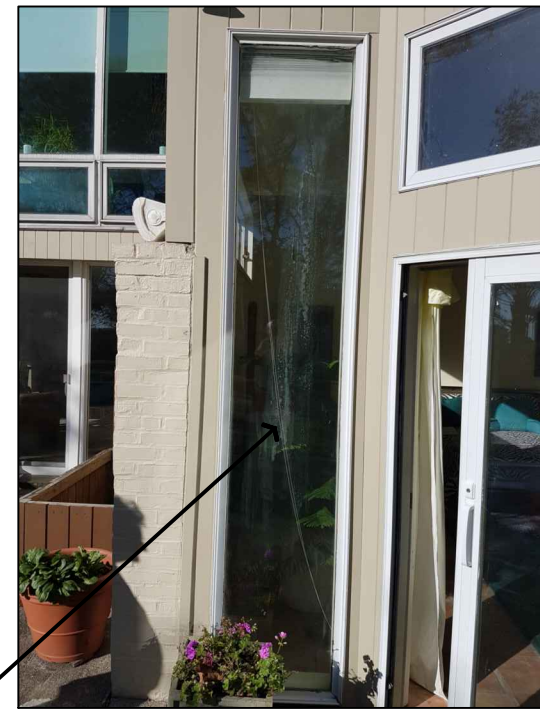
REPLACE INSULATING GLAZING UNIT IN BEDROOM 101 (EXTERIOR VIEW) [ref. Keynote 2]
