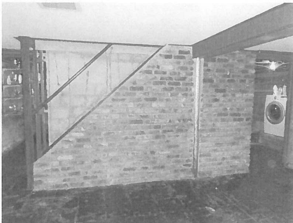
Basement ACM Black Floor Mastic
