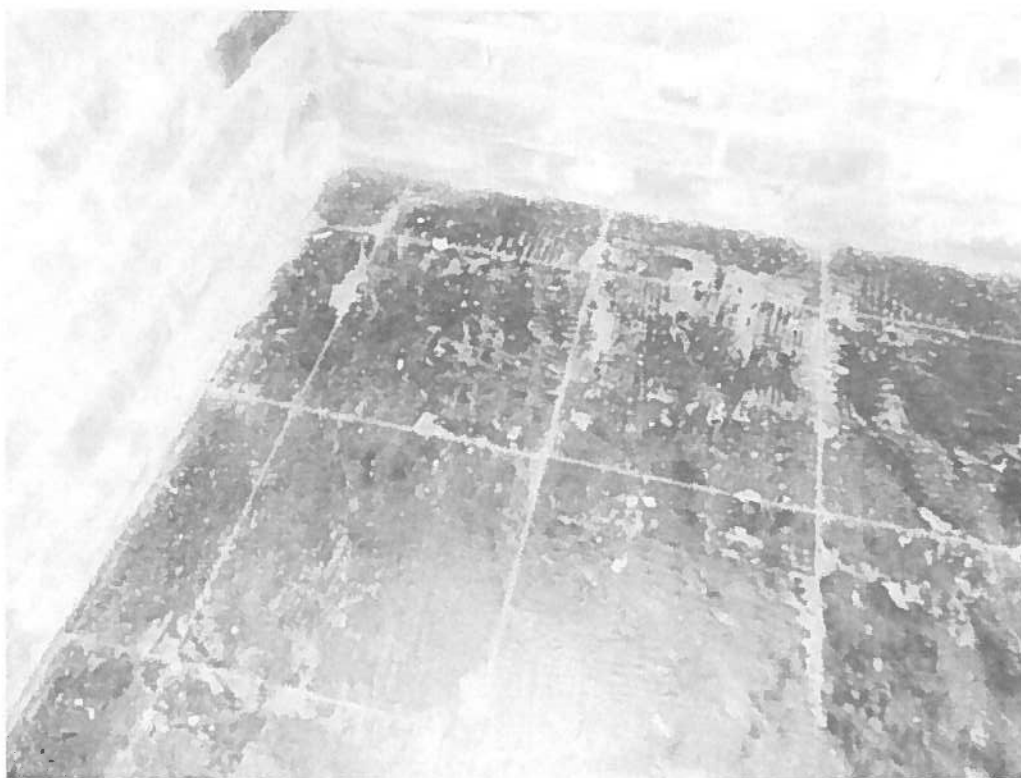
Basement ACM Black Floor Mastic
