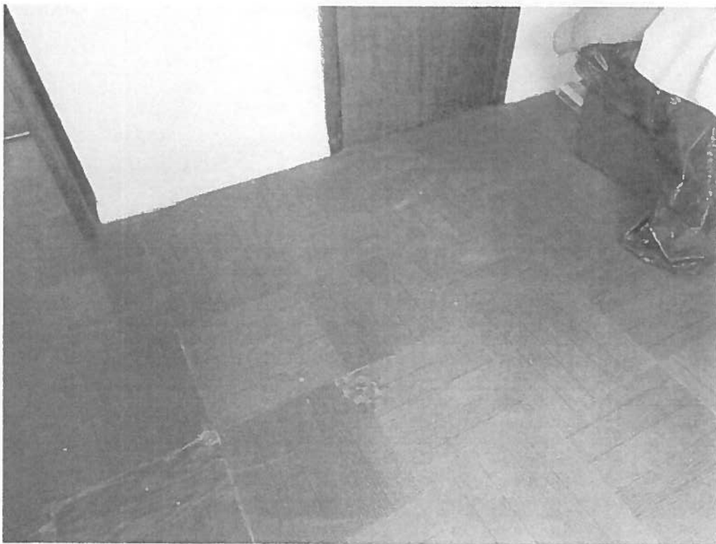
2 nd Floor ACM Brown Self-Stick Floor Tile
