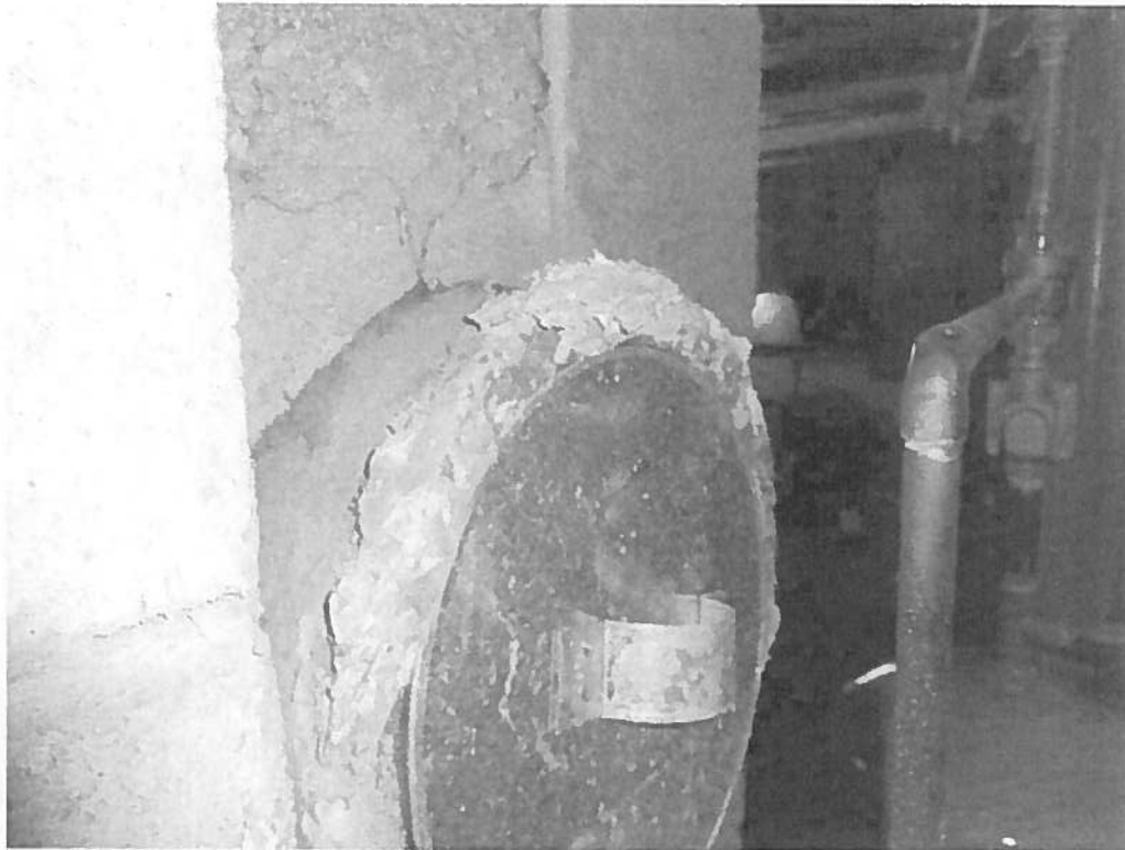
ACM Chimney Flue Cement
