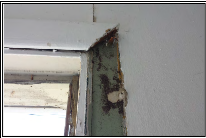
Photograph 7 Mold behind entryway trim
