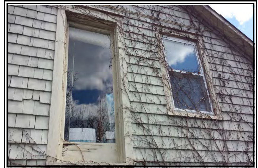
Photograph 4 Window with ACM glazing
