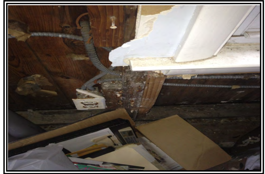
Photograph 8 Mold on wooden frame in kitchen
