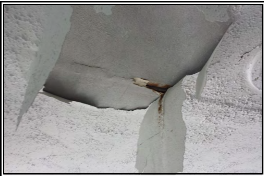
Photograph 3 Textured ceiling containing ACM
