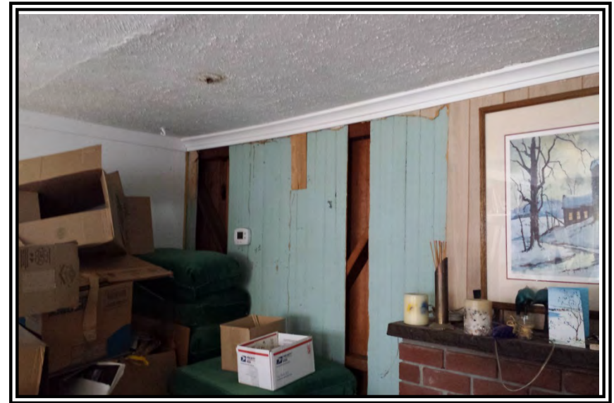
Photograph 2 Lead-containing blue paint behind wood paneling
