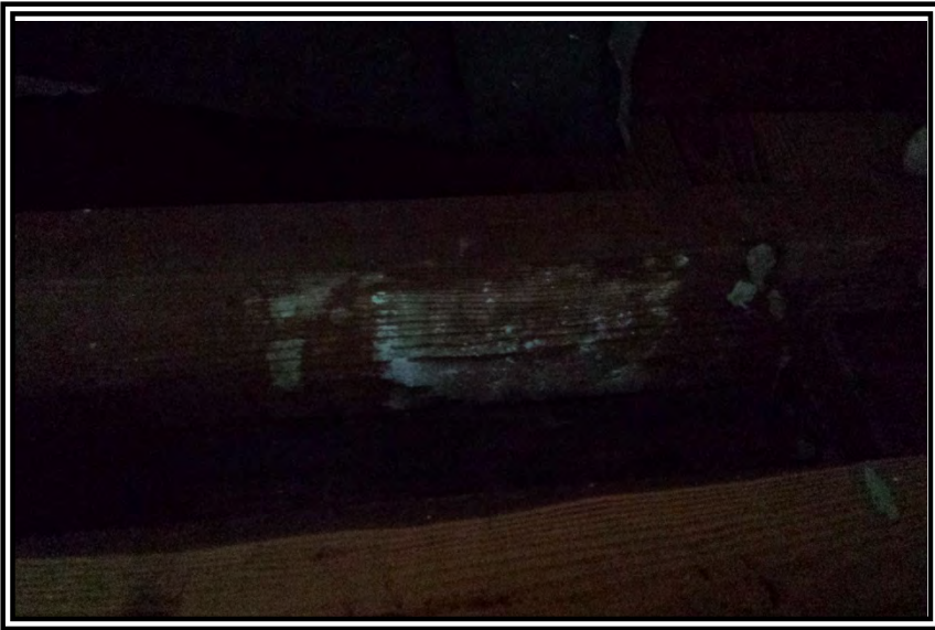
Photograph 5 Mold on wood closet frame opposite stairs
