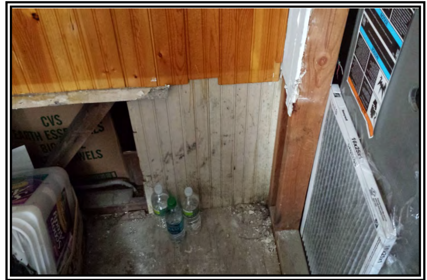
Photograph 6 Mold on wood paneling adjacent to furnace
