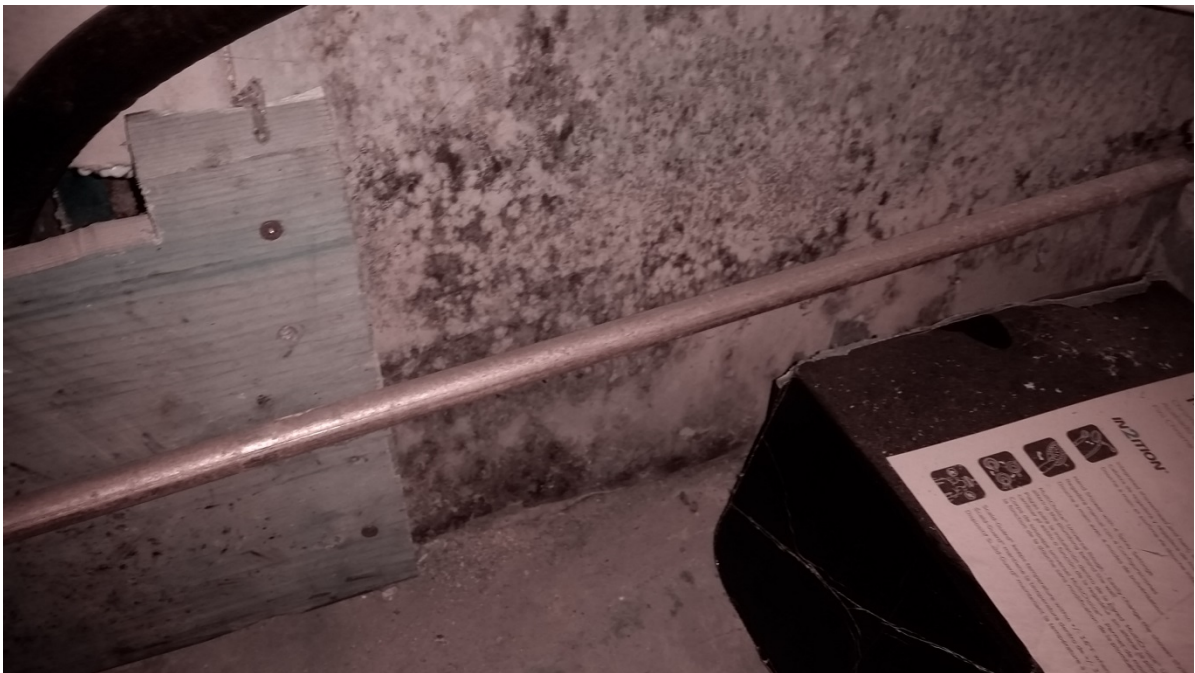
Mold Growth on Wall behind Heating Unit in Garage
