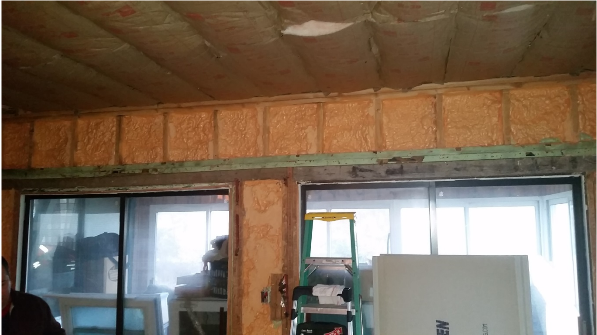
Green Lead Paint on Wood Wall Frames
