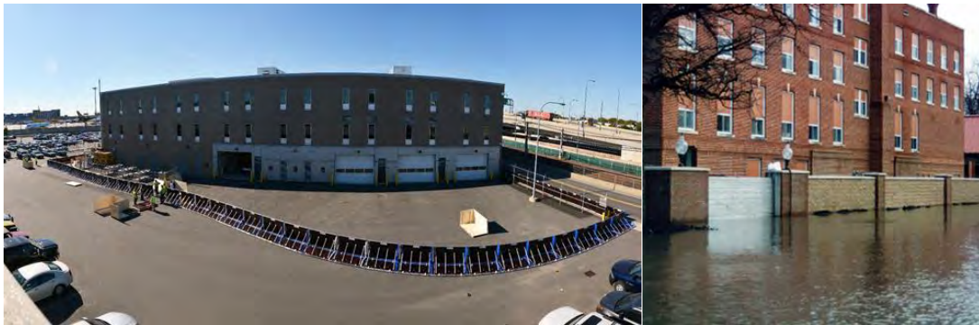
Figure 45 - Temporary Flood Panels (left) and Flood Wall with Temporary Flood Gate (right)
