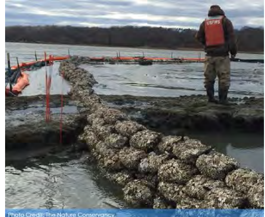
Figure 35 - Examples of Thin-Layer Deposition (left) and Oyster/Clam Shell Bags for Marsh Edge Protection (right)
