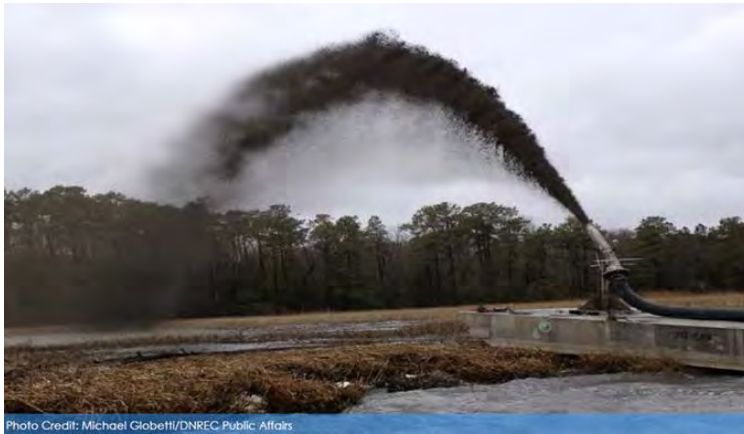
Figure 35 - Examples of Thin-Layer Deposition (left) and Oyster/Clam Shell Bags for Marsh Edge Protection (right)
