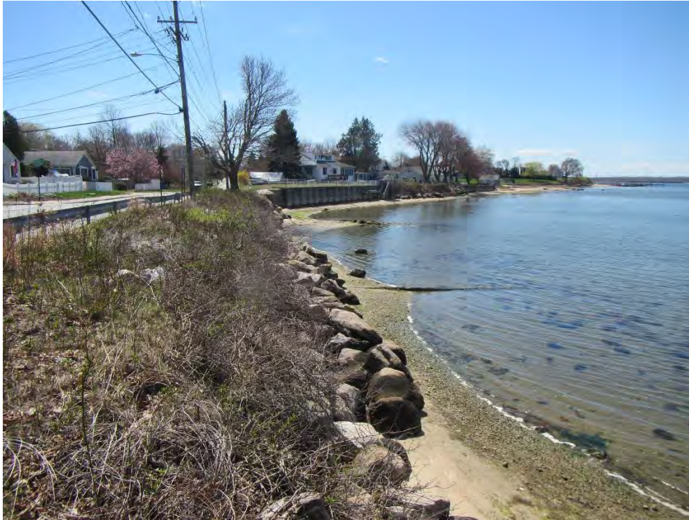
Figure 19 - Seawall and Stone Revetment along Niantic River Road
