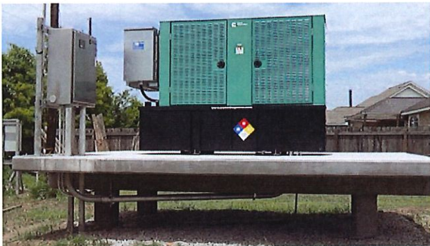
Figure 64: Example of a Generator (Elevated to Protect Against Flooding)
