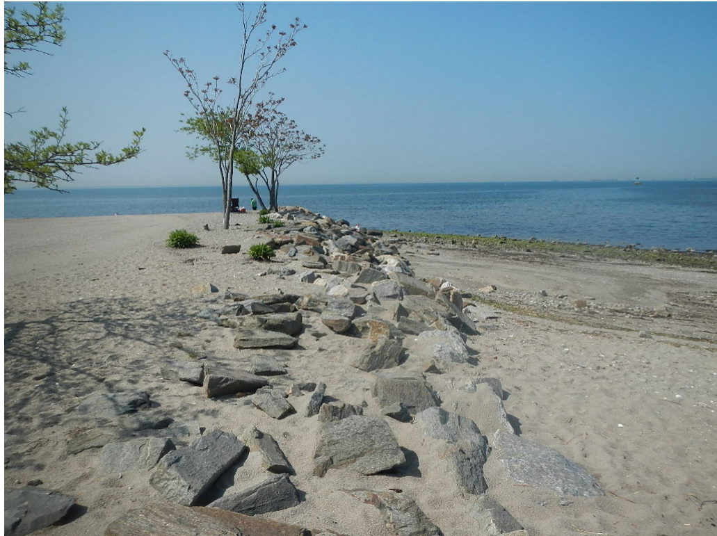
Photo 4: Existing Groin Area May 2016
