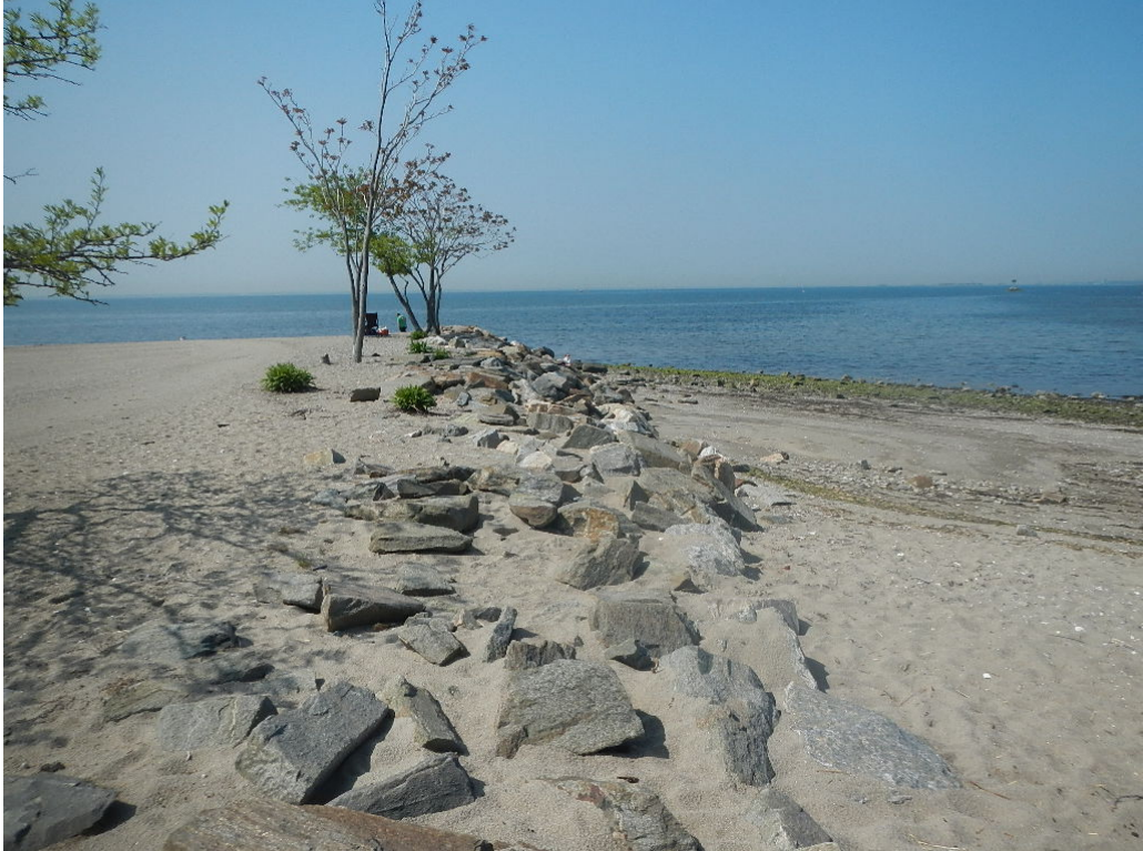
Photo 4: Existing Groin Area May 2016
