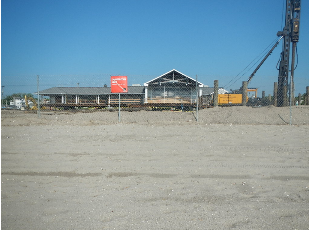
Photo 4: Construction Area May 2016
