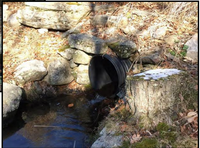
Photo No. 97 (Upstream above, downstream right)
