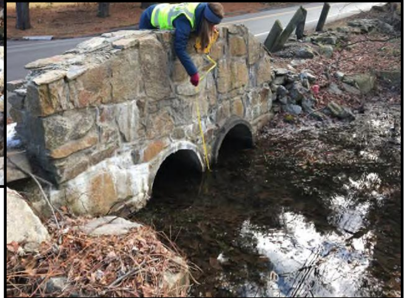
Photo No. 71 (Upstream above, downstream right)
