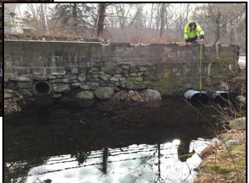
Photo No. 72 (Upstream above, downstream right)
