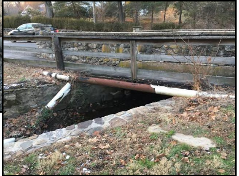
Photo No. 25 (Upstream above, downstream right)
