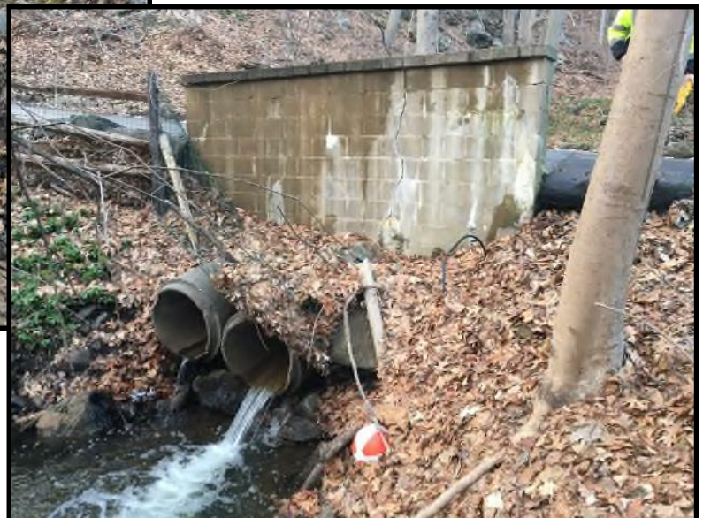
Photo No. 59 (Upstream above, downstream right)
