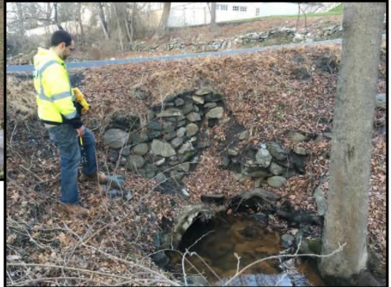
Photo No. 58 (Upstream above, downstream right)
