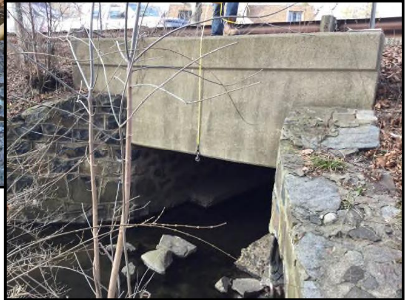
Photo No. 31 (Upstream above, downstream right)
