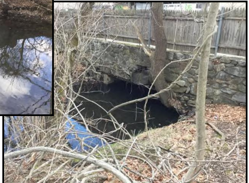
Photo No. 32 (Upstream above, downstream right)
