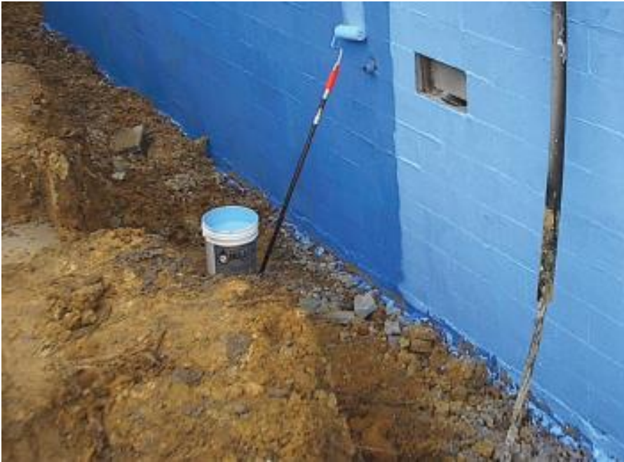
Figure 4-11: Application of Waterproofing (FEMA, 2013)
