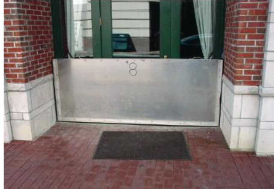
Figure 4-10: Aluminum door flood shield used for flooding less than 3 feet deep. (FEMA, 2013)
