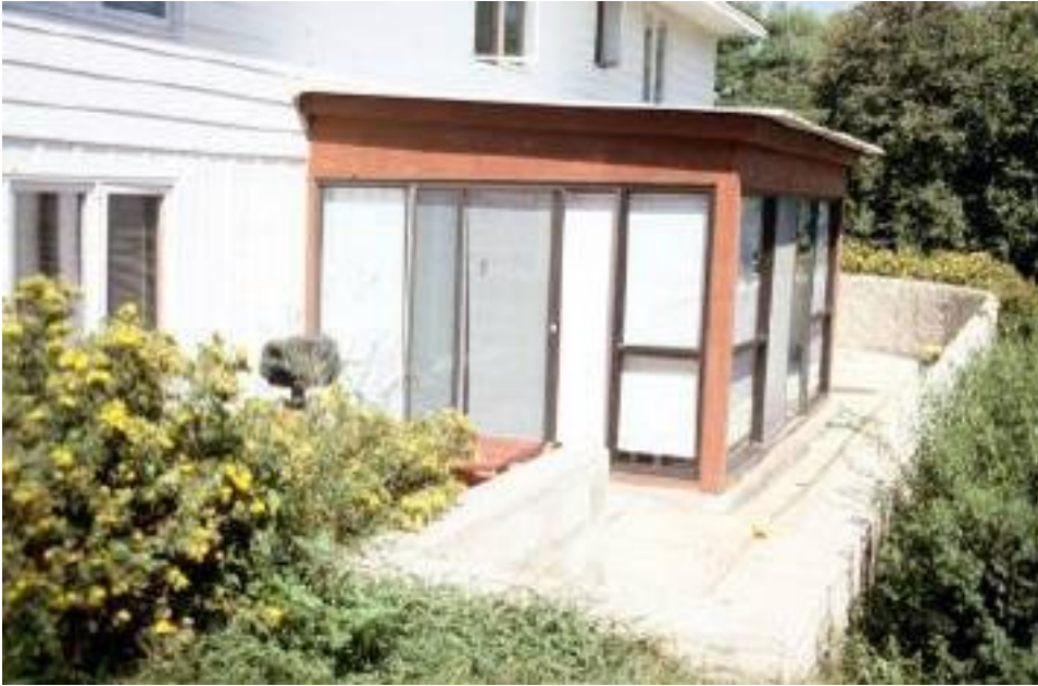
Figure 4-9: Structure protected by a floodwall (FEMA, 2007)
