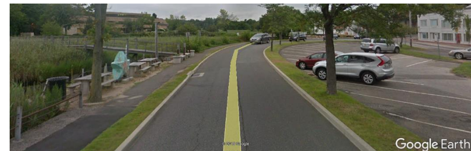
Figure 3.21: Images showing shoreline structures within Coastal Flood Inundation Areas along Parker Harding Plaza
