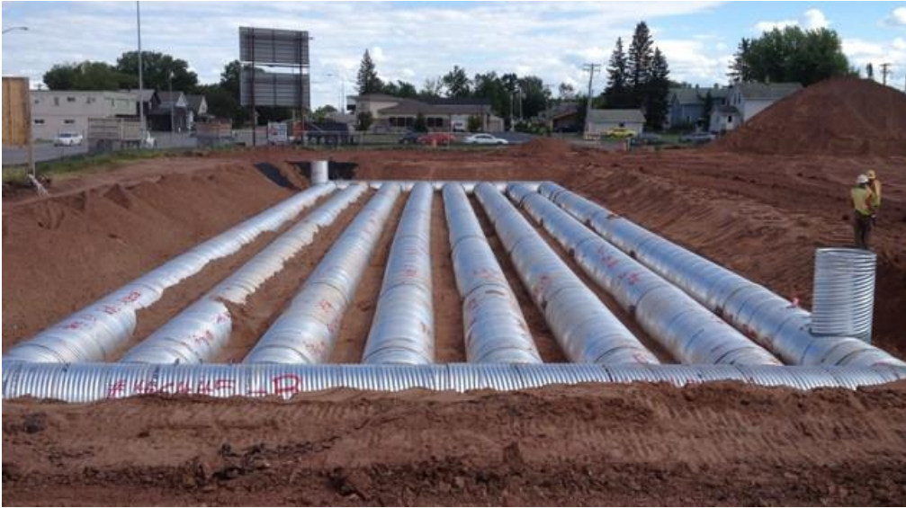
Figure 4-4: Underground stormwater detention; photo from Contech Figure Engineered Solutions
