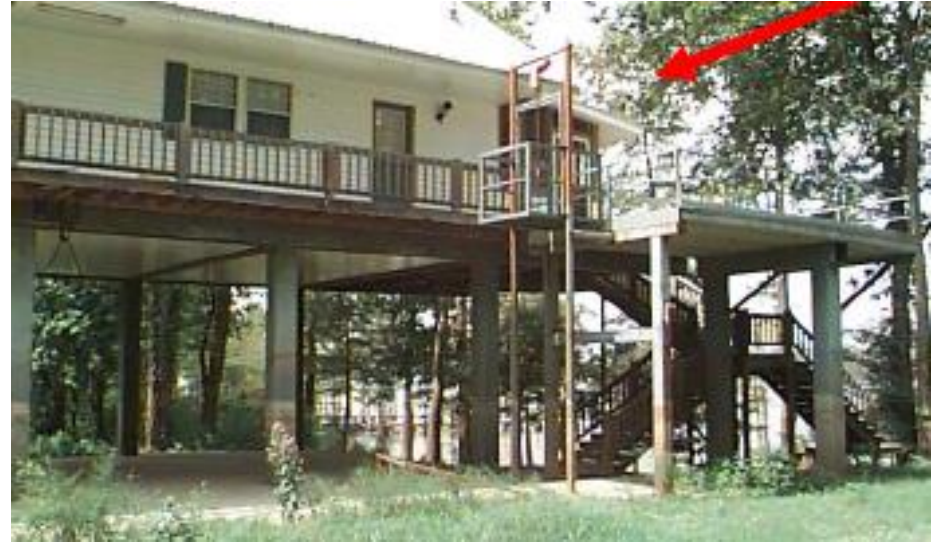
Figure 4-12: Elevating Structures (FEMA, 2013)
