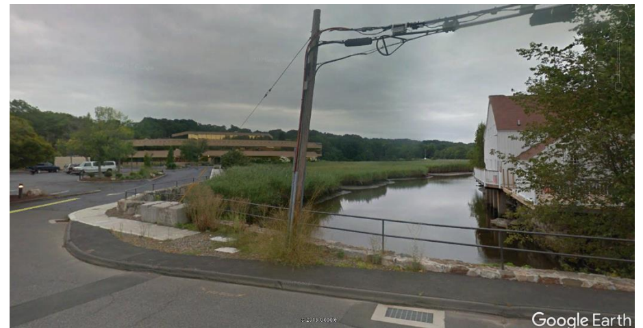
Figure 3.20: Images within Coastal Flood Inundation Areas near Gorham Island Road
