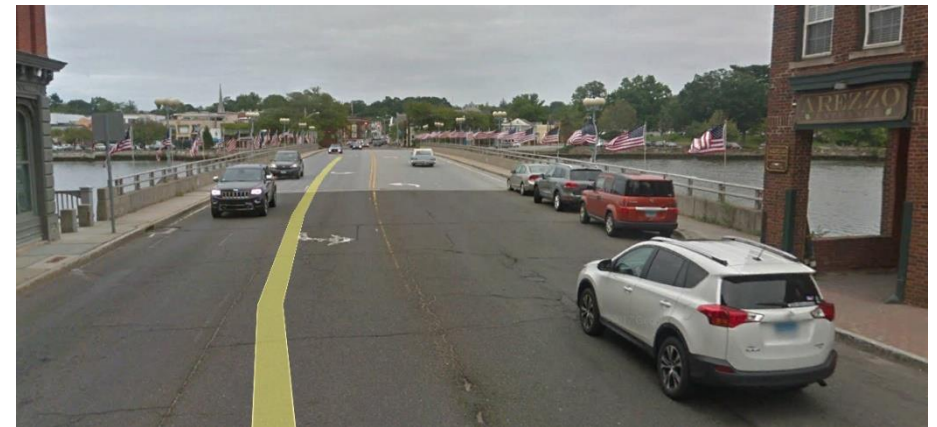
Figure 3.23: Images of the Bridge, looking east from Wilton Road
