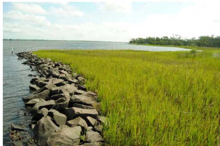
Hybrid living shoreline with rip rap. Image credit: Jesse baud, living shoreline , https://www.flickr.com/photos/151809992@N06/37911236174 , (CCO 1.0).
