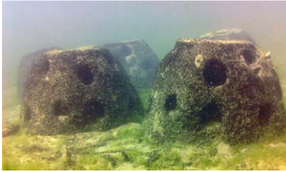
Rip rap or oyster reefs located just offshore of a marsh help to reduce the energy of waves hitting the coastline. Hollow concrete reef balls provide a manmade structure with functions similar to rip rap but designed to act as habitat for local fish and invertebrates. Under the right conditions, reef balls may encourage the establishment of oysters leading to an oyster reef. Photo credit: Reef Balls at Dutch Springs by Neil DeMaster, (CC BY-ND 2.0). https://www.flickr.com/photos/84169650@N07/10544449634 .
