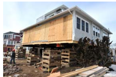
A home is elevated Photo: Shoreline Times
