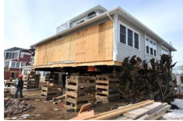
A home is elevated Photo: Shoreline Times
