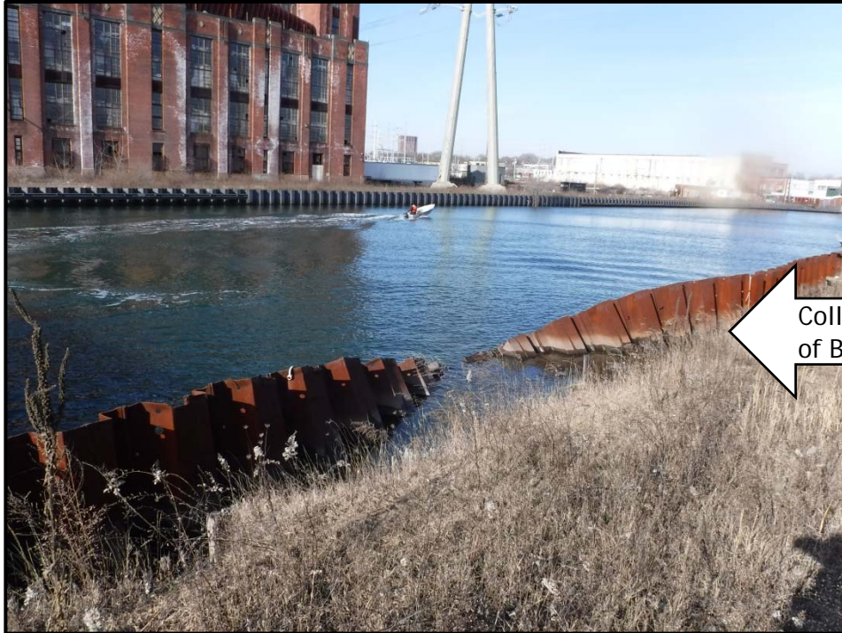
Photo No. 13: Steel sheet pile bulkhead along Gateway Terminal, looking northwest, photo taken January 8, 2016.
