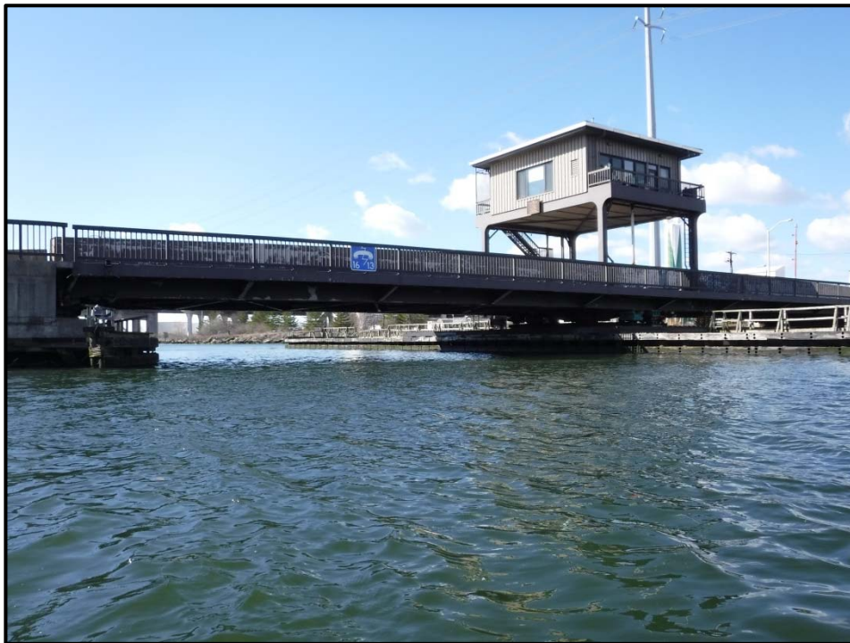
Photo No. 4: Chapel Street Bridge, looking south, photo taken March 18, 2016.
