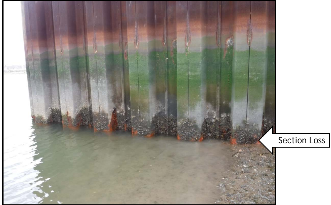
Photo No. 3: Bulkhead for United Illuminating Utility Pole, looking south, photo taken on March 18, 2016.
