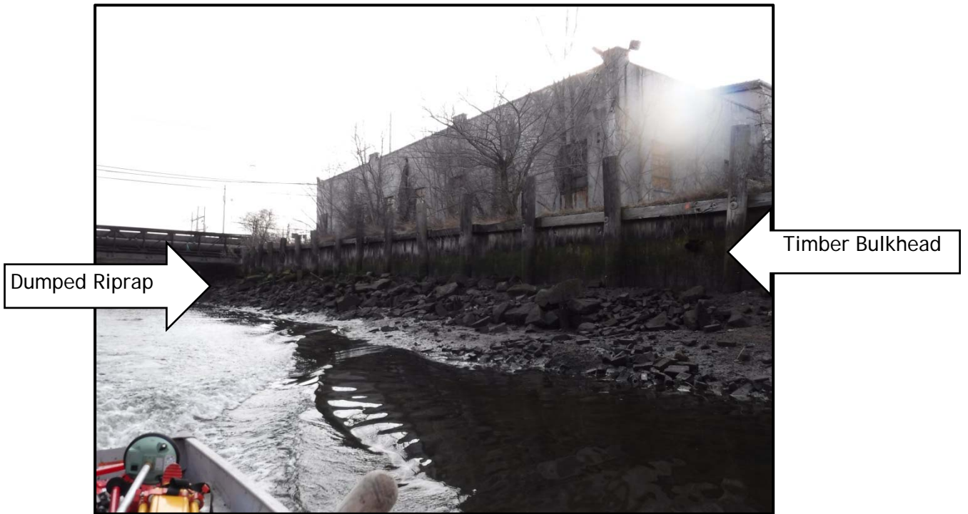
Photo No. 30: Timber bulkhead with riprap at toe along former St. Gobain, looking southwest, photo taken February 19, 2016.
