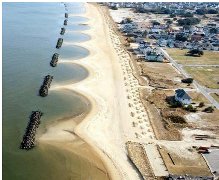
Figure 8: Example of offshore breakwaters with dune feature.
