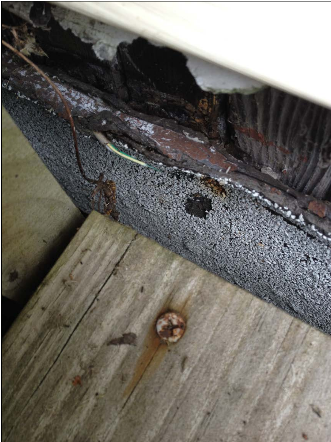
Exterior between staircase and house – a bead of tar sealer (to seal two layers of rolled roofing together) (Reddish tinted material only on perimeter of the sheets)
