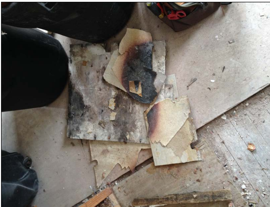
Living room floor near waste barrels – scrap linoleum pile
