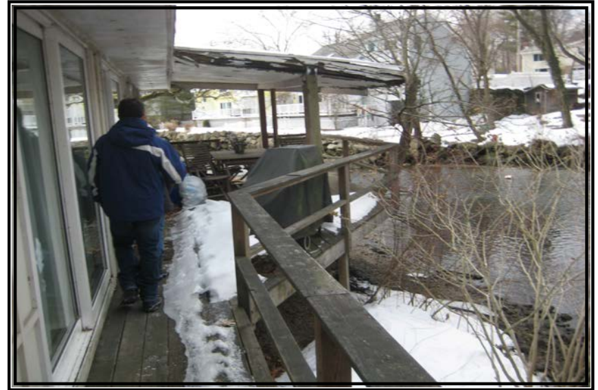
Photograph 2 Deck overhanging watercourse
