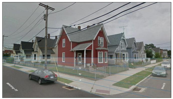
Figure 9 - Intersection of Whiting Street and Broad Street with elevation markers for raised street
