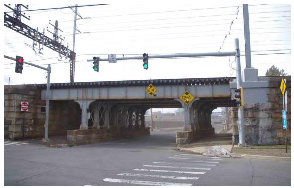
Photograph 64. Broad Street Railroad Bridge, viaduct stone retaining walls and catenary structures, camera facing north.
