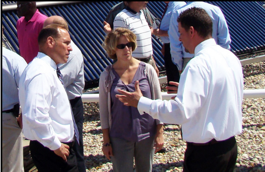
South District Administrator Michael Lajoie (L), and Deputy Commissioner Cheryl Cepelak listen to Plant Facility Engineer 1 Joseph Suchecki explain the solar hot water system installed on the roof of building 9A at York CI.
