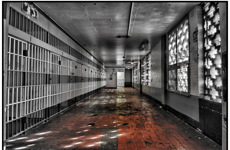
Plant Facilities Engineer I, Jay Harder's award winning photograph of Bridgeport Correctional Center's old North Wing prior to renovation.
