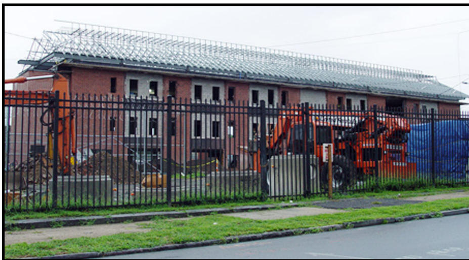
Bridgeport Correctional Center's Old North Wing undergoes extensive renovations
