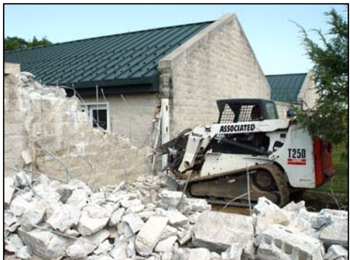
Building Envelope Integrity Remediation Project in progress.
