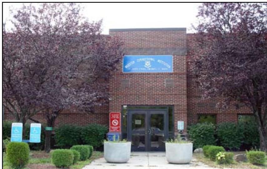
Front entrance of the closed Webster facility.
