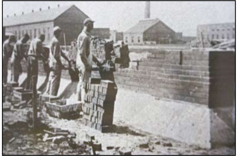
Inmates from the old Wethersfield State Prison work on constructing the perimeter walls of the Cheshire Correctional Institution which opened in 1910.
