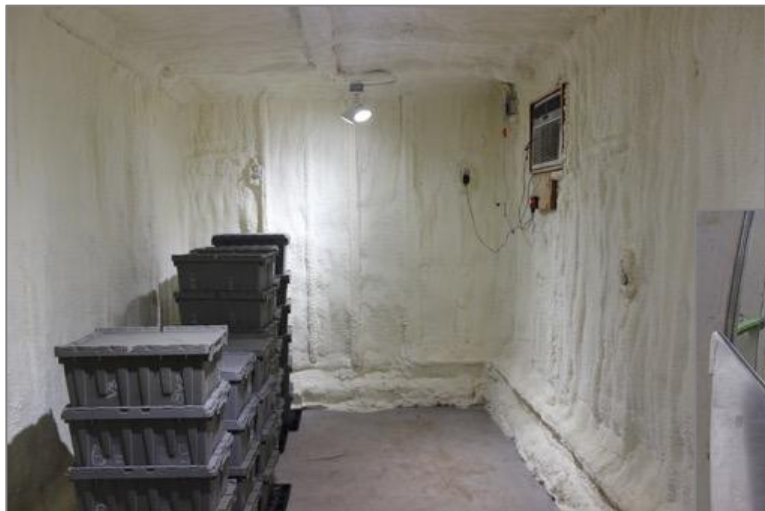
Photo: National Center for Appropriate Technology
