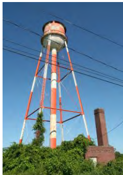
Existing Water Tower
