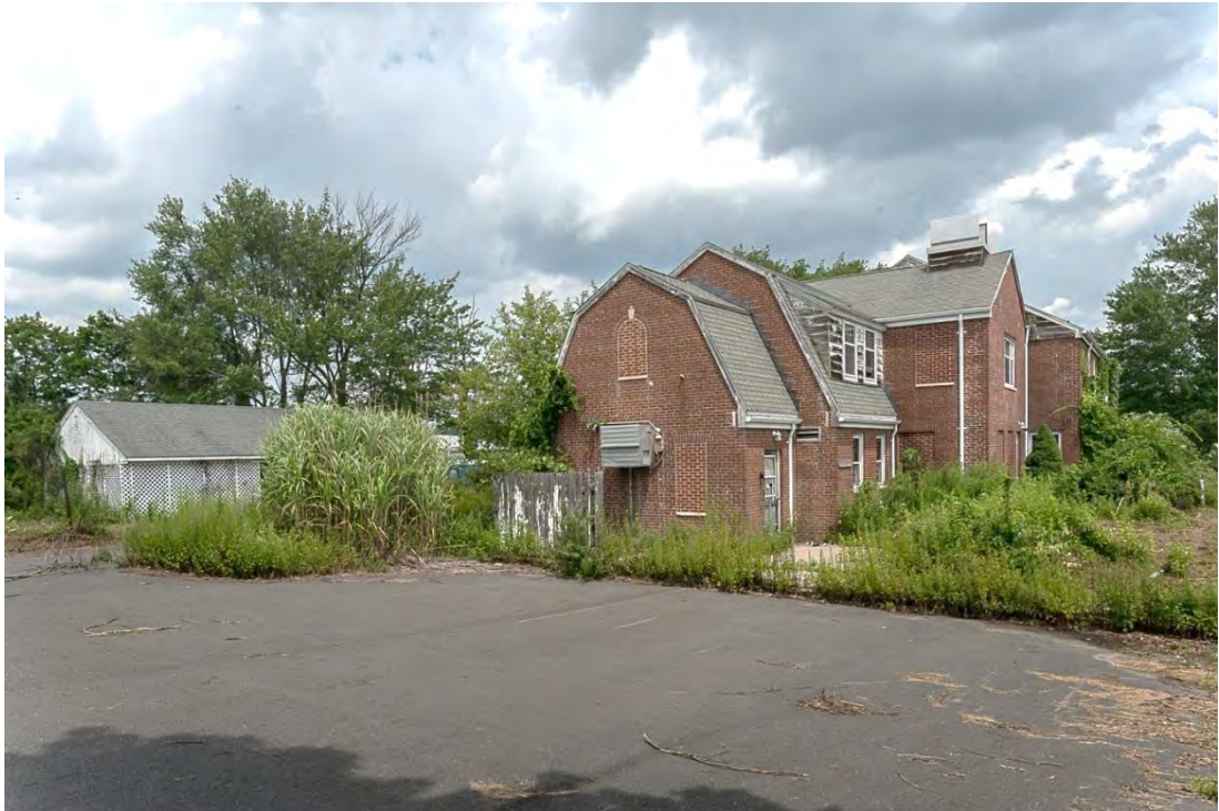
Photo 23. Building 4, view northeast showing covered patio, west elevation and part of façade.
