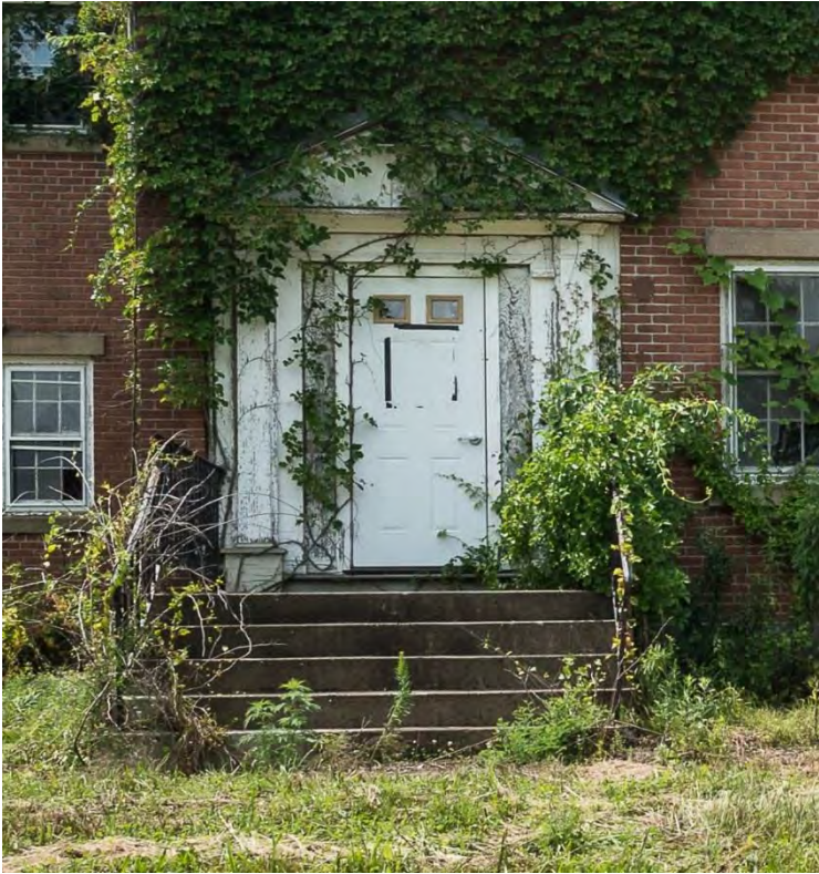
Photo 2. Building 1, view northeast showing main entrance.
