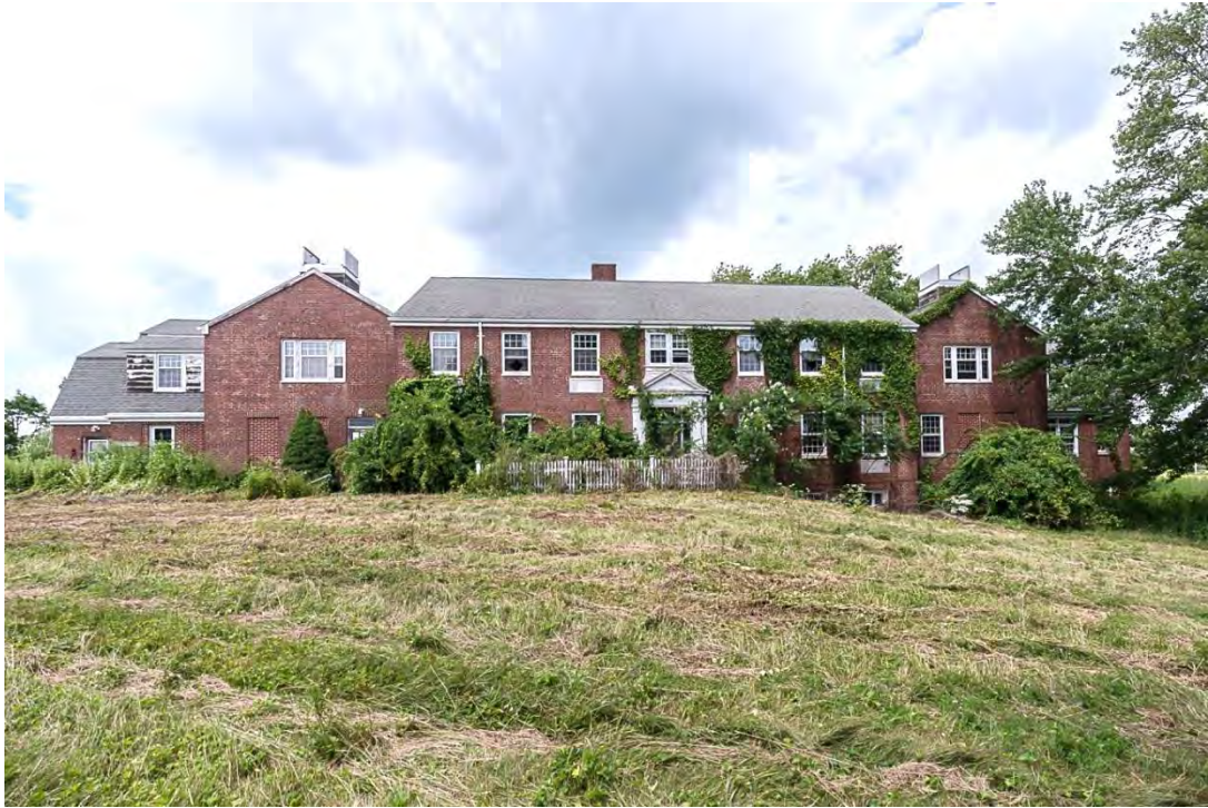
Photo 21. Building 4, view northwest showing façade.
