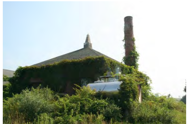
Reference Photo: West Elevation with Milk Storage Tank
