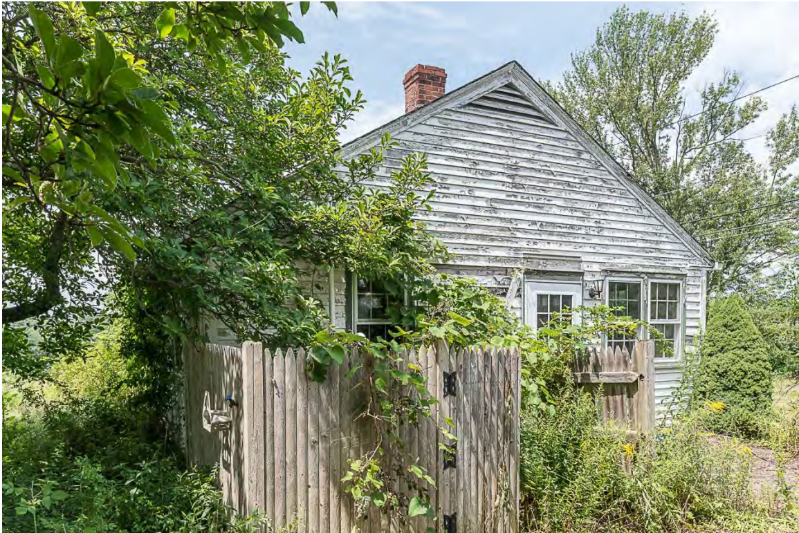
Photo 15. Building 2, view west showing façade.
