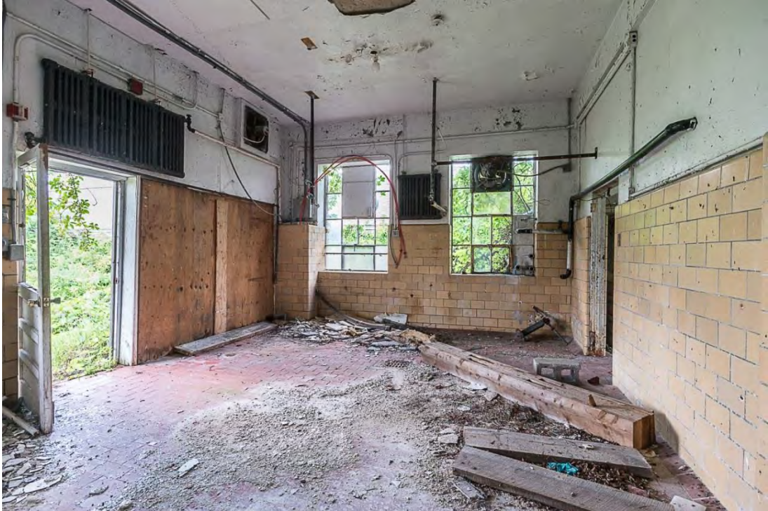
Photo 37. Building 7, interior view north showing west room.
