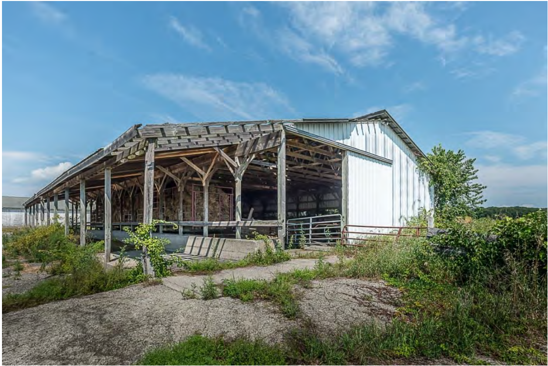
Photo 44. Building 10, view northwest showing south and east elevations of heifer barn.
