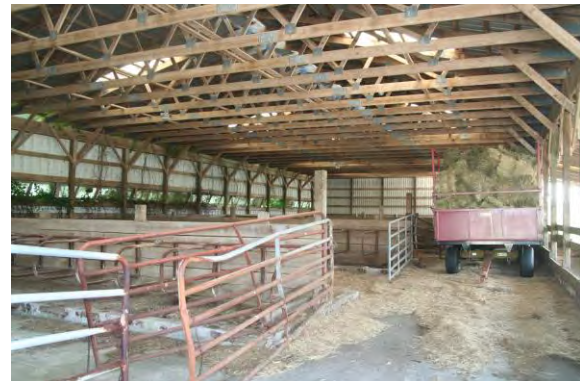
Interior #1 Looking East
