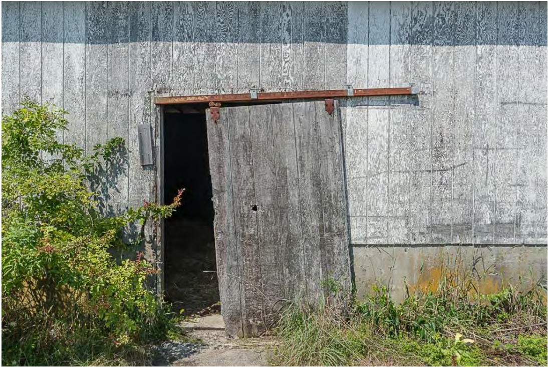
Photo 40. Building 9, view west showing original door on east elevation
