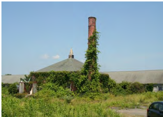
Reference Photo: South Elevation
