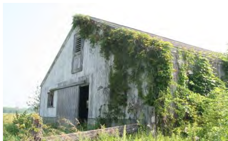
Reference View of North Elevation
