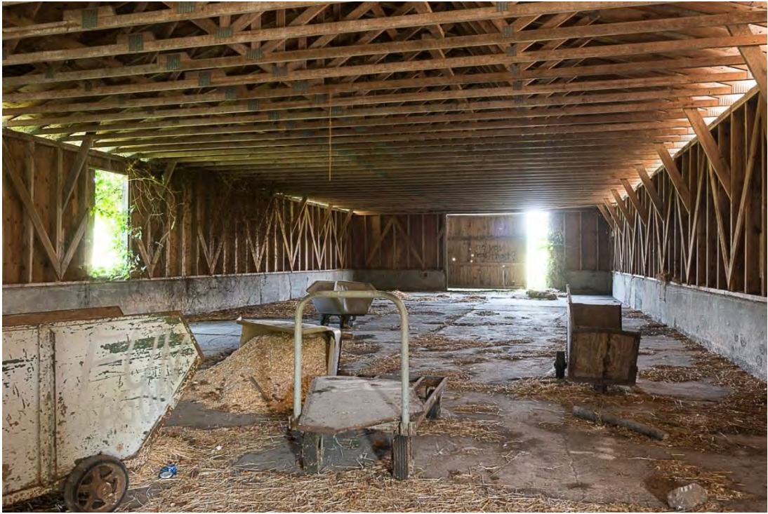
Photo 41. Building 9, interior view north.
