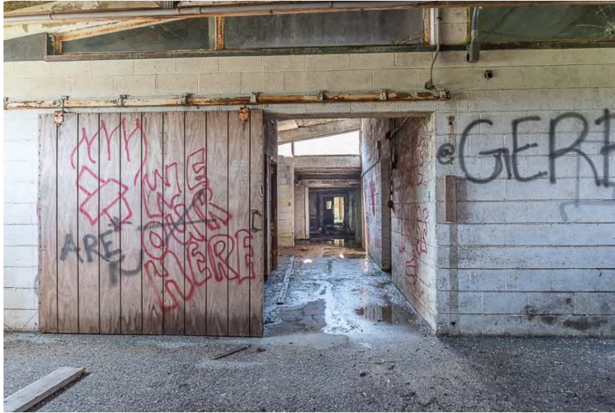
Photo 41. Building 9, interior view south showing entrance to corridor to milking barn.
