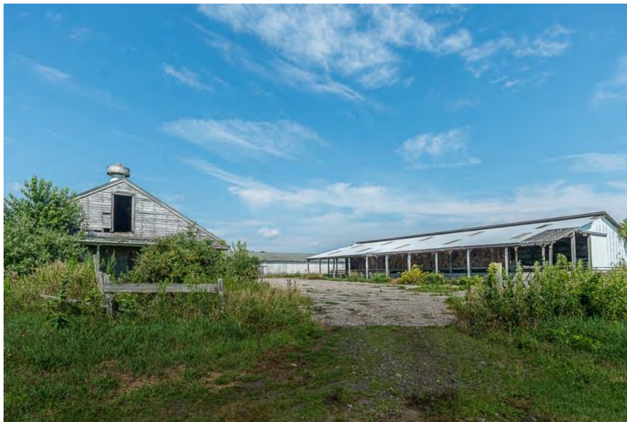
Photo 42. Building 10, view northwest showing east elevation of milking barn, east elevation of hay barn and south elevation of heifer barn.
