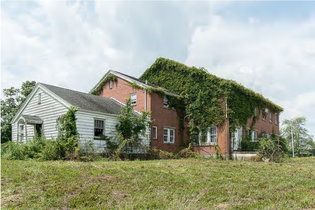
Photo 5. Building 1, view southwest showing east and north elevations.
