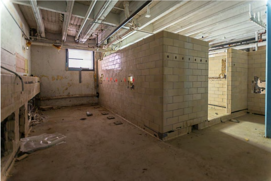
Photo 12. Building 1, basement interior view southeast showing tile enclosure.
