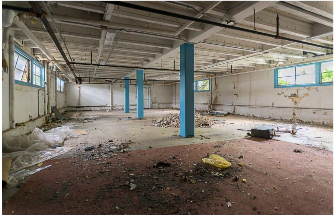
Photo 13. Building 1, basement interior view southeast.
