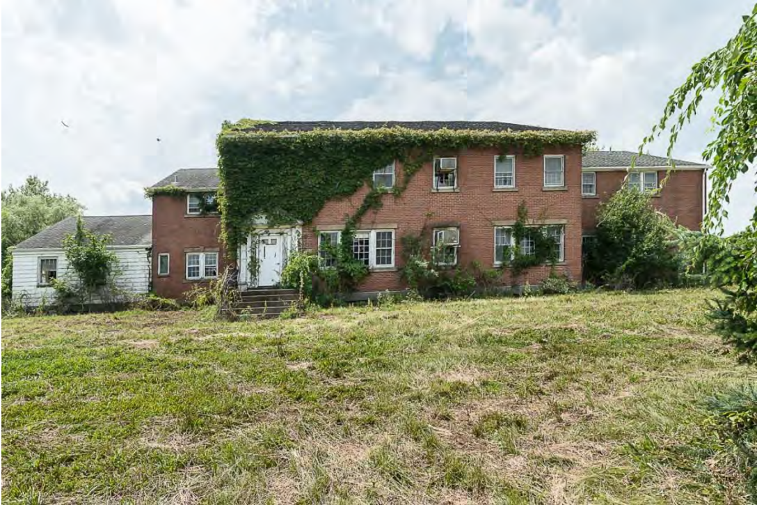
Photo 1. Building 1, view northeast showing façade.
