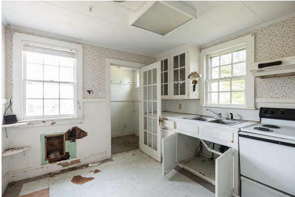
Photo 19. Building 2, interior view southwest showing kitchen.
