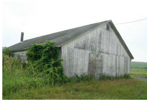
View Looking Northeast - Hydraulic Equipment Lifted Roof
