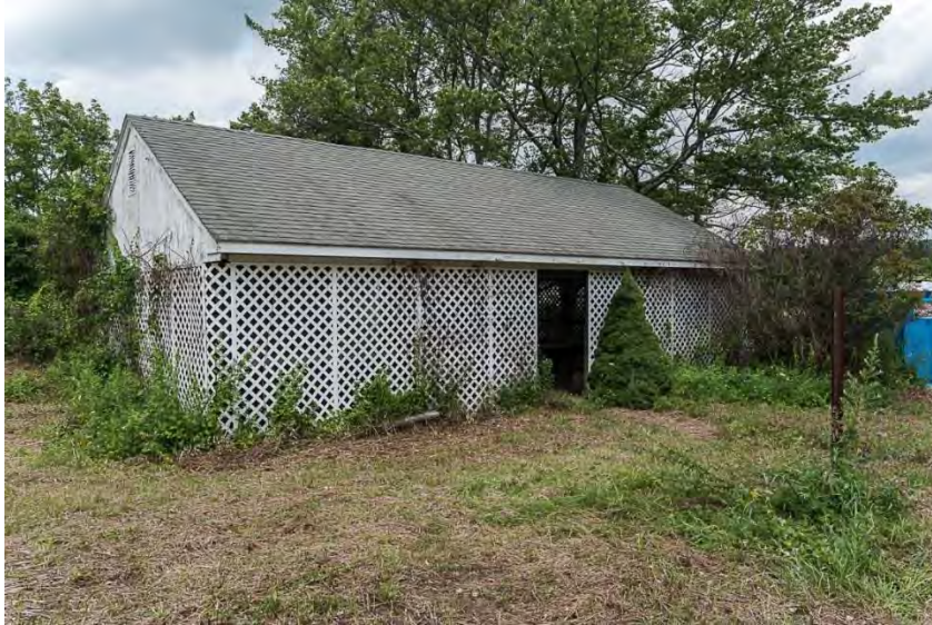
Photo 31. Building 5 view northeast showing west and south elevations.
