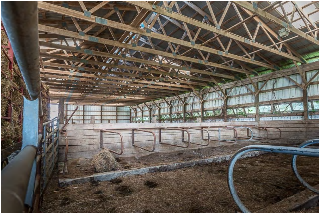
Photo 45. Building 10, interior view northwest showing roof trusses and open stalls.
