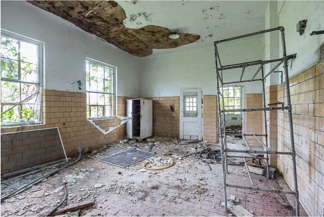
Photo 36. Building 7, interior view south showing east room.
