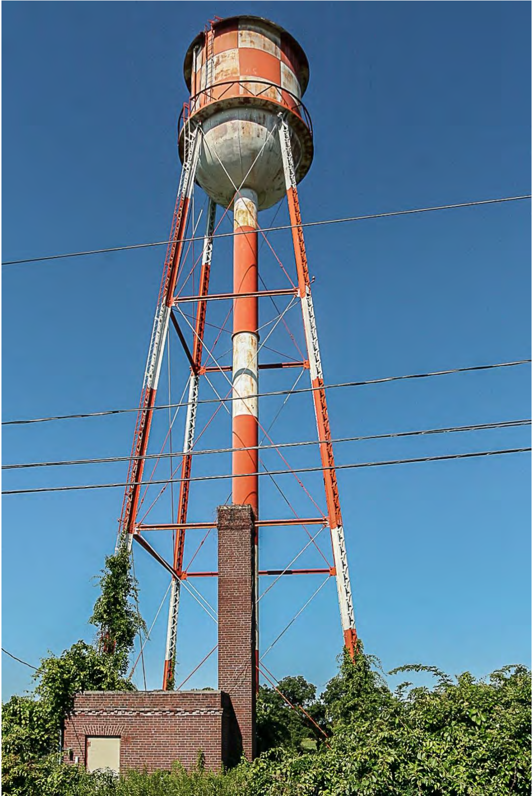
Photo 47. Water tower and pump house, view north.
