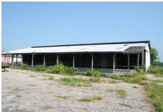
South Elevation of Heifer Barn Looking North from Barn Yard
