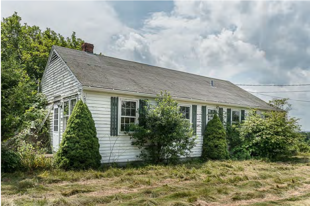
Photo 14. Building 2, view southwest showing façade and north elevation
