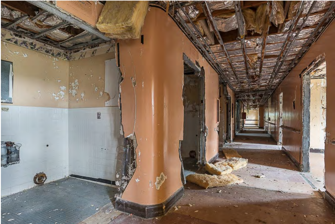
Photo 28. Building 4, second floor interior view northwest showing corridor.
