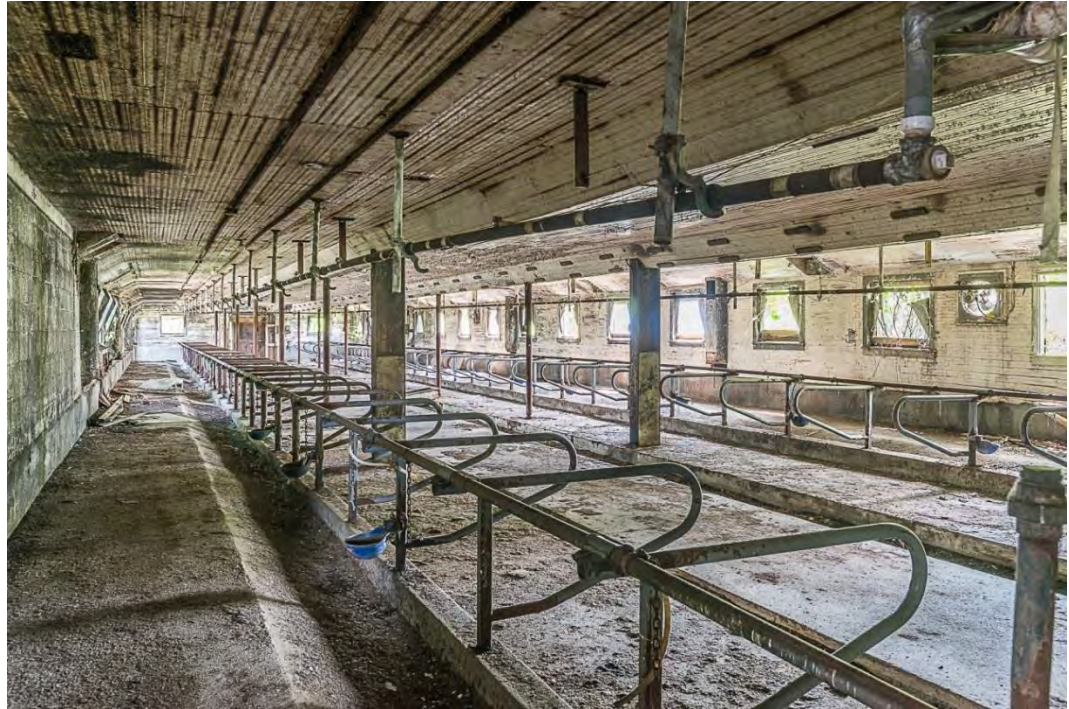
Photo 38. Building 8, interior view southeast showing concrete floor and open stalls
