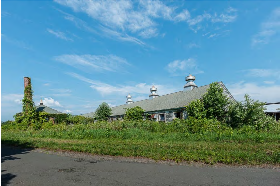
Photo 34. Building 7 view northwest showing milk house and dairy barn.
