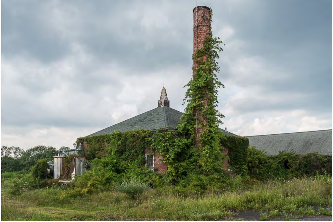
Photo 35. Building 7, view northwest showing milk house and chimney.
