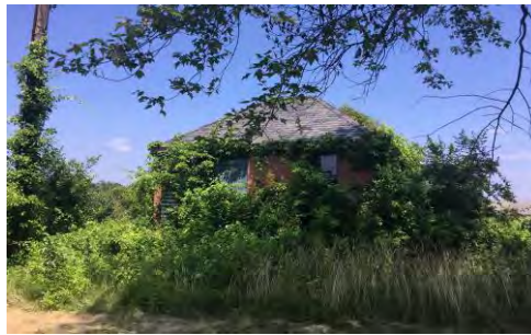
View Looking West from Barn Access Road
