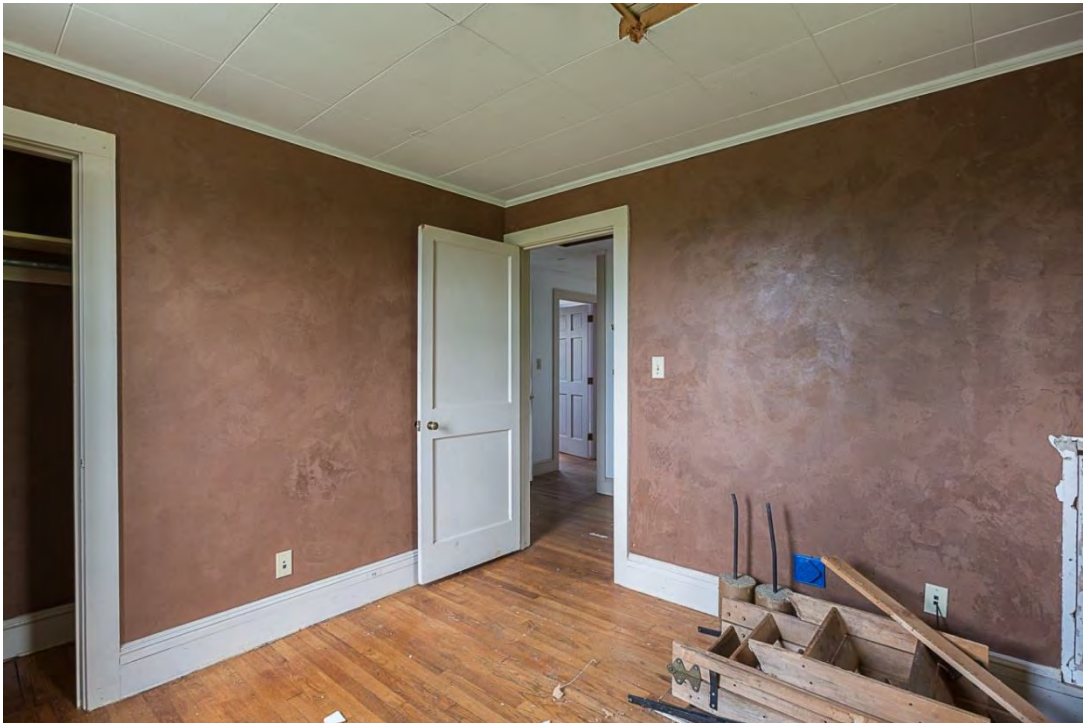
Photo 18. Building 2, interior view southwest showing bedroom.
