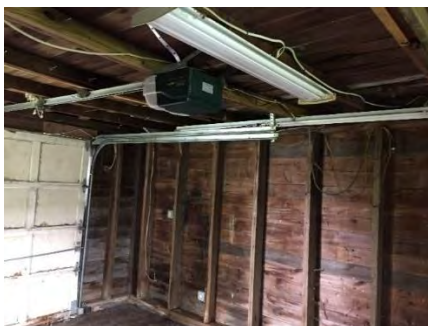
Building 3: Photo of interior wood framing.
