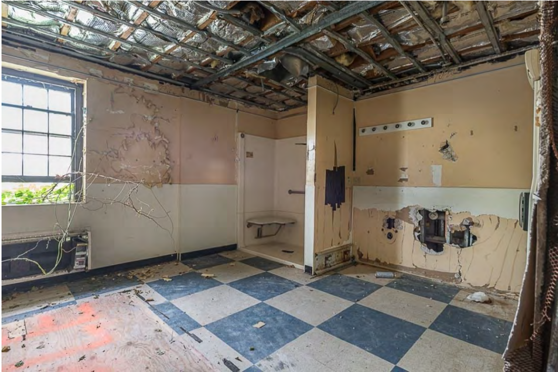
Photo 29. Building 4, second floor interior view northeast showing therapy room.
