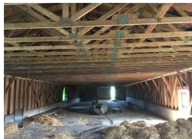
Reference View of Interior Looking North
