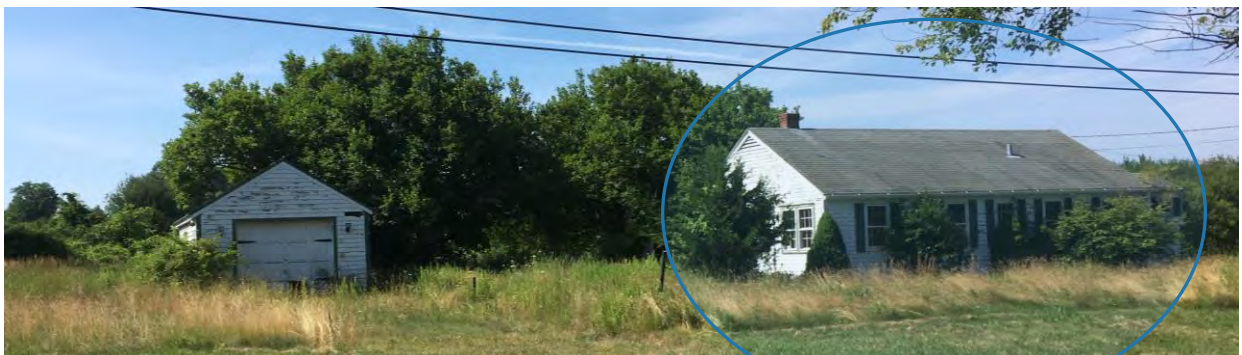
North Elevation Showing Building #2 FOREMAN'S HOUSE and Building #3 DETACHED GARAGE
