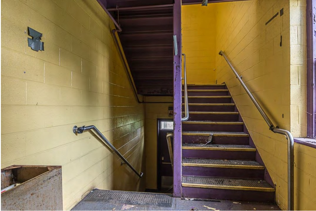
Photo 30. Building 4, first floor interior view northwest showing steel stairs.
