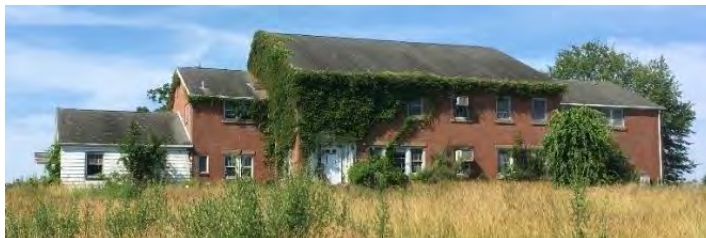
Reference Photo: North Elevation
