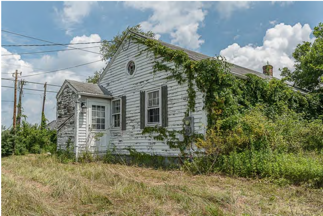
Photo 17. Building 2, view northeast showing west elevation.
