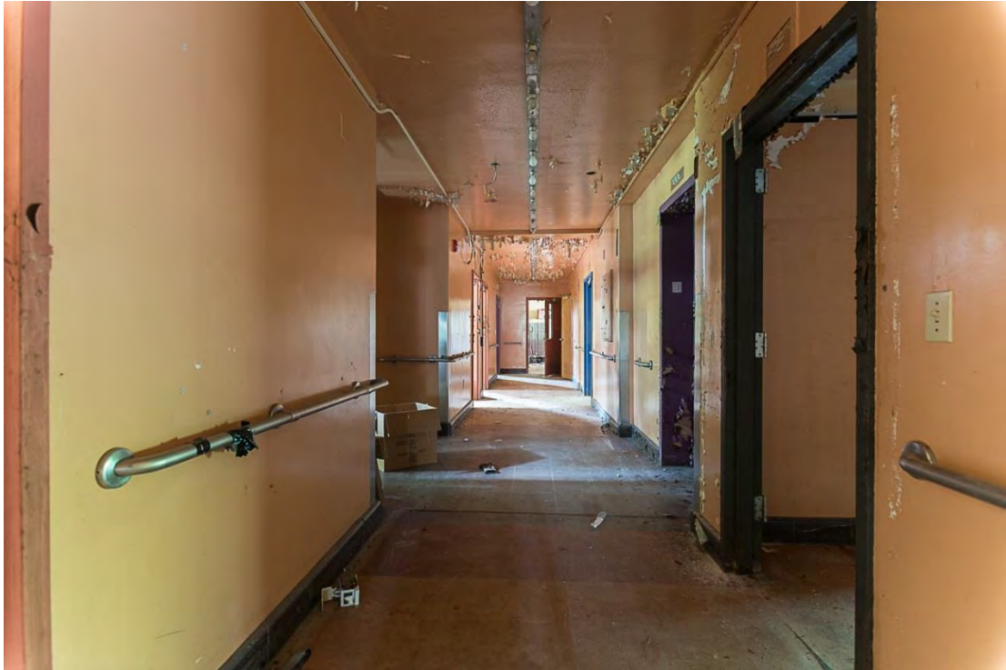
Photo 26. Building 4, first floor interior view southwest showing corridor.
