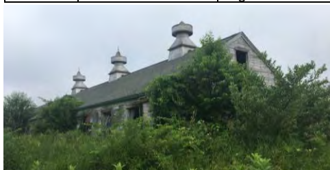
Reference Photo: West End of Dairy Barn Looking Southeast
