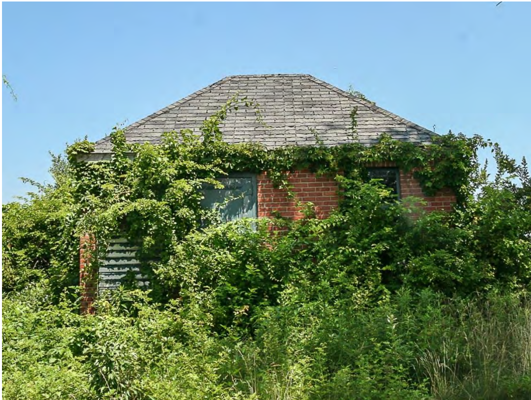
Photo 32. Building 6, exterior view north showing facade.
