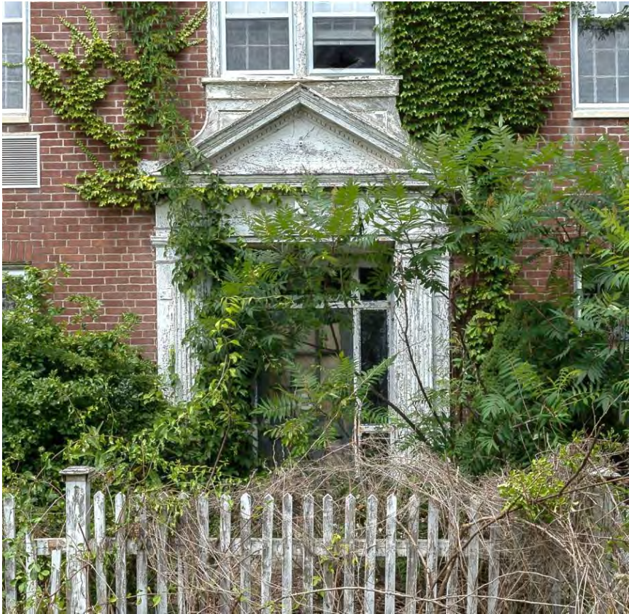
Photo 22. Building 4, view northwest showing main entrance with Georgian elements.
