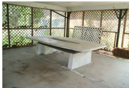
Interior View of Patio & Concrete Plant Potting Table
