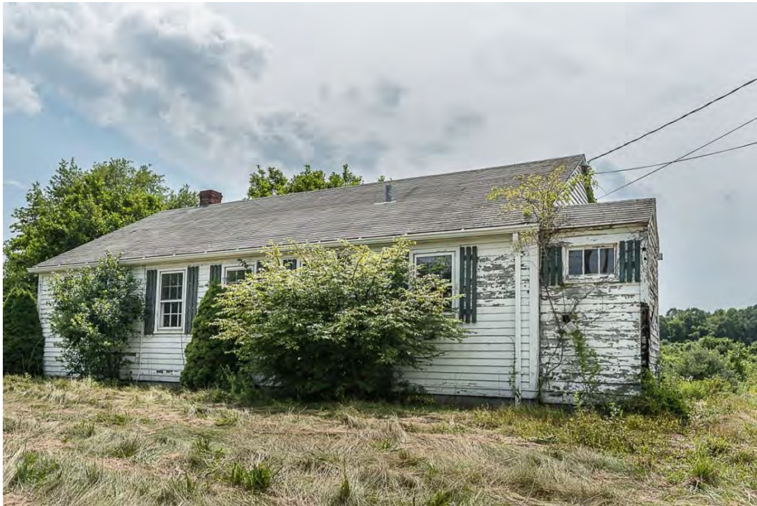
Photo 16. Building 2, view south showing north elevation.
