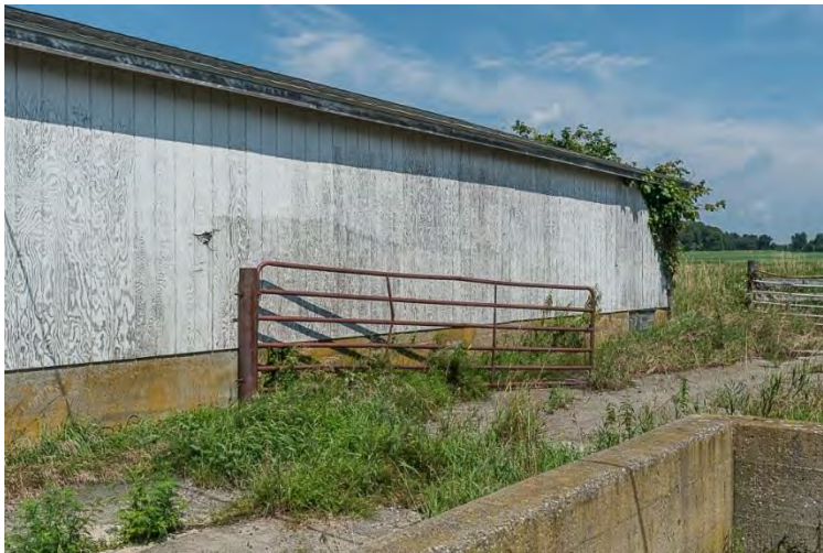
Photo 39. Building 9, view northwest showing east elevation.
