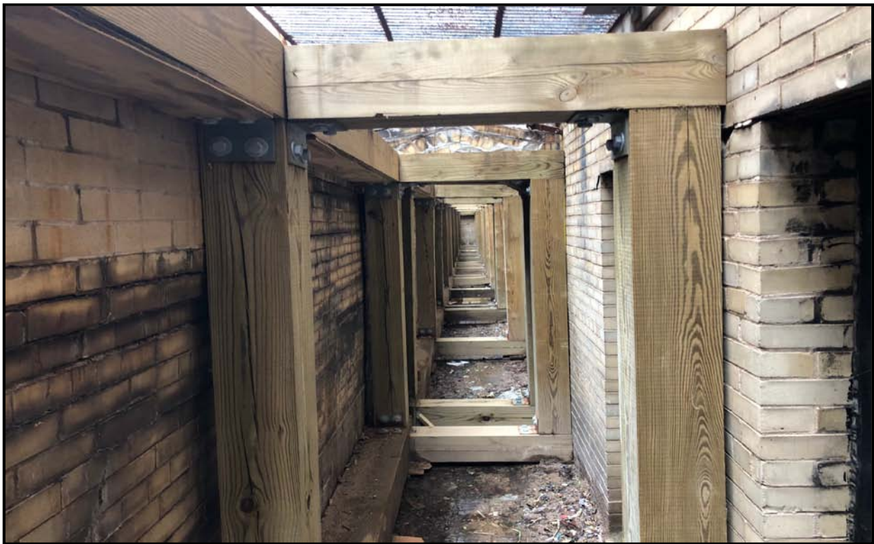
PHOTO 2 – South Areaway Timber Shoring
