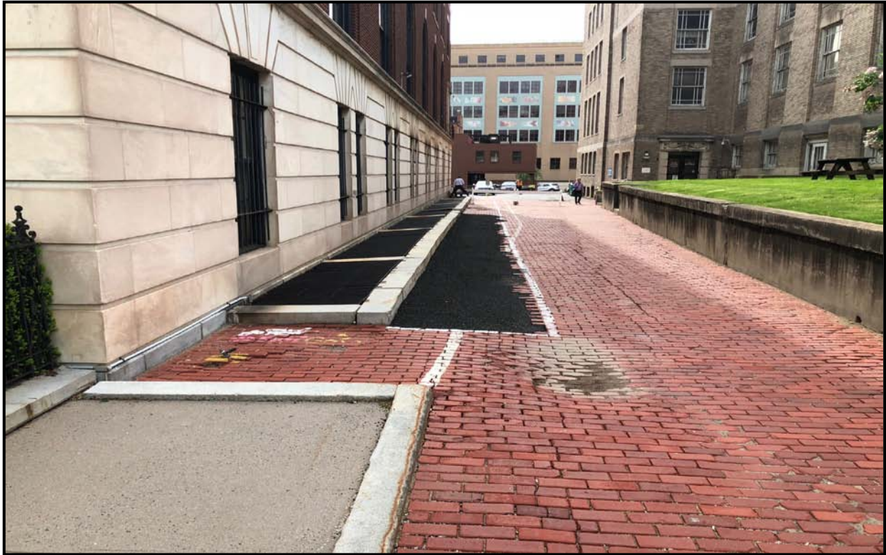
PHOTO 1 – South Alley Way Looking East.
