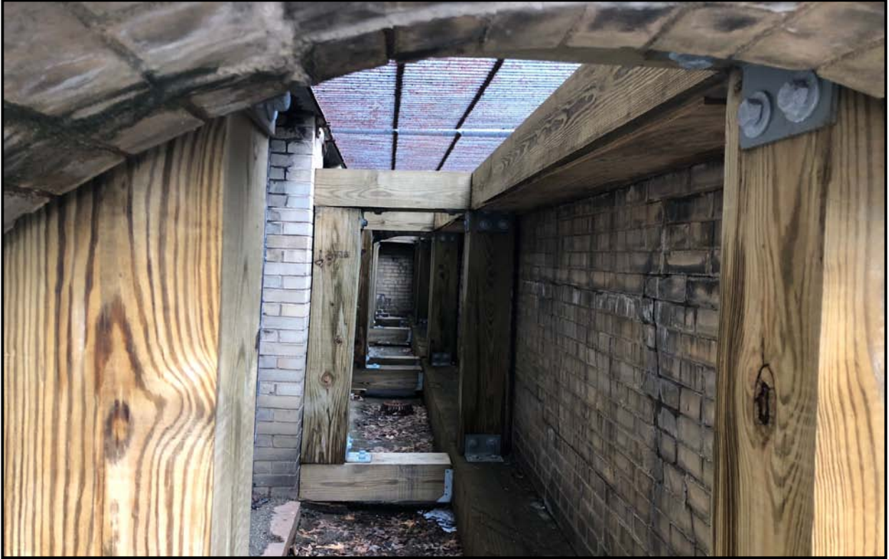
PHOTO 3 – North Areaway Timber Shoring
