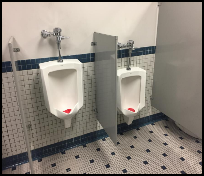
Exhibit "M2" Toilet Plumbing Fixtures
