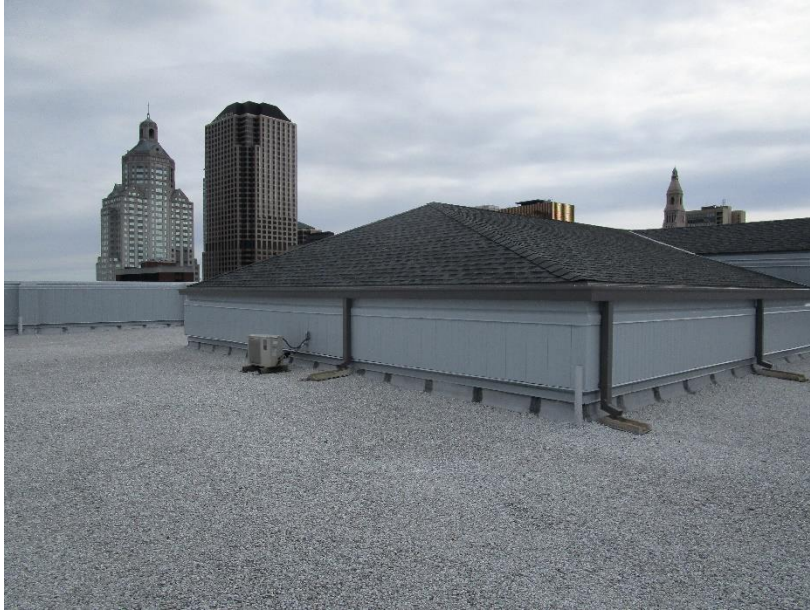
Figure 103. Asphalt shingle roofing and aluminum wall panels at mechanical penthouse.
