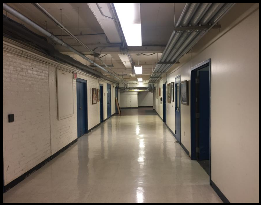
Exhibit "E7" Basement Corridor Lighting
