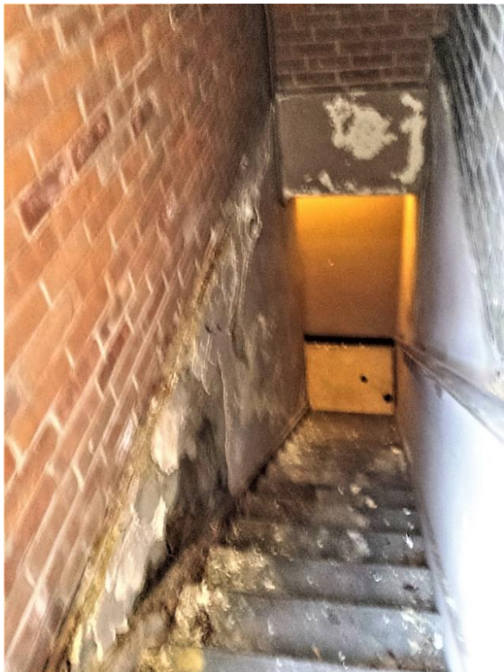
Figure 36. Interior of stair bulkhead at 20 Trinity Street.
