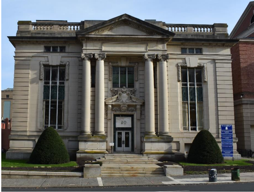
Figure 1. West façade at 20 Trinity Street. Historic photographs of this elevation indicate the doors and windows present were not part of the original construction.
