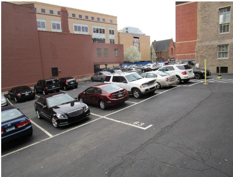
Figure 108. Bituminous asphalt surface at parking lot behind 18 Trinity Street.
