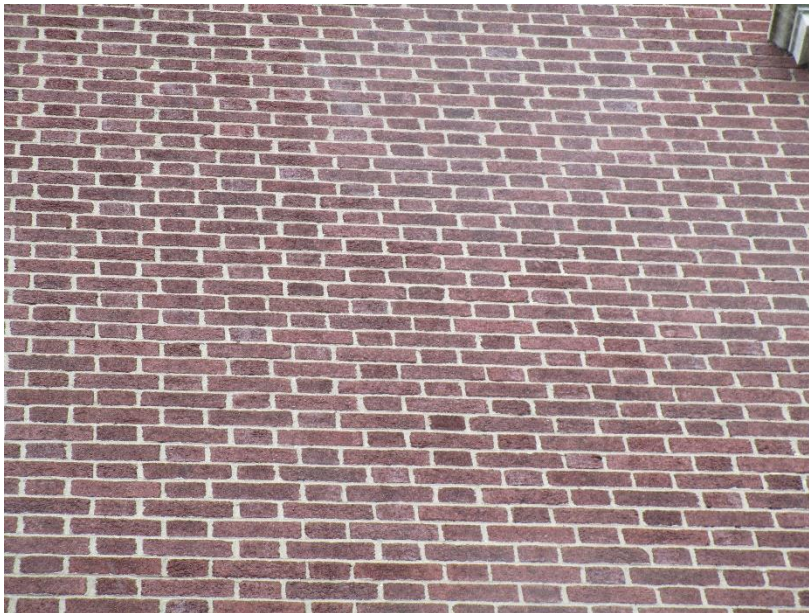
Figure 88. Mortar in brick joints at 30 Trinity Street.
