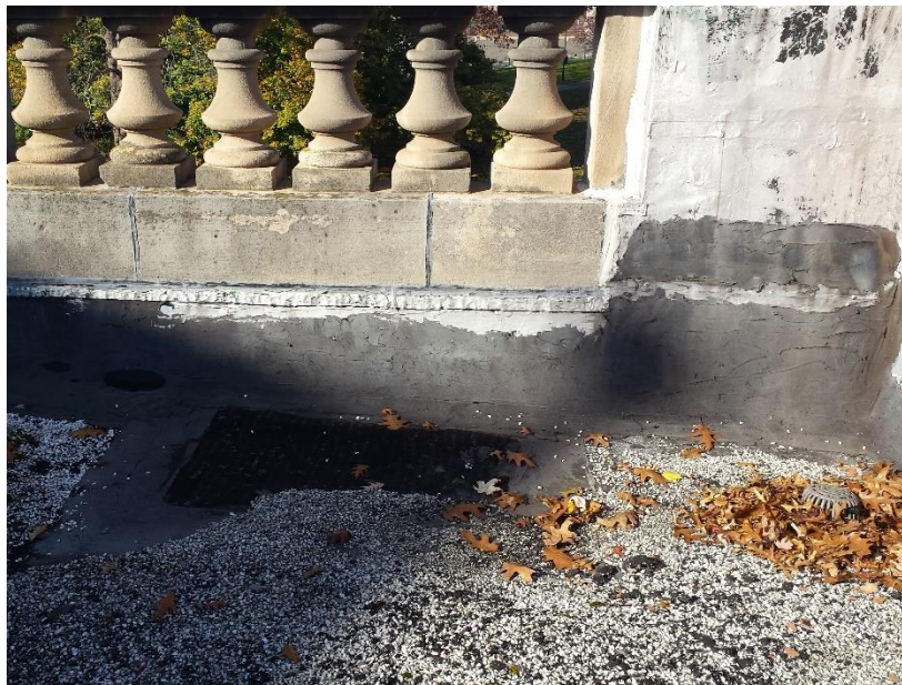
Figure 30. Roofing mastic applied to repair the base flashing.
