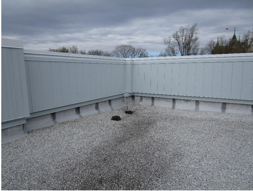
Figure 101. Wall panels at roof parapet and roof drains.
