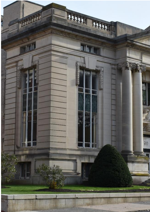
Figure 21. Windows at the northwest corner of 20 Trinity Street.
