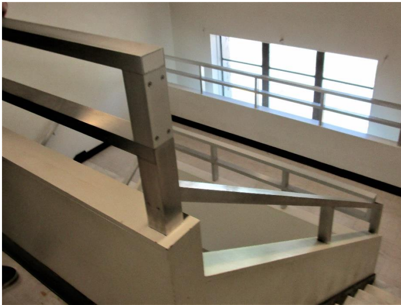
Figure 115. Guard and handrails at west stair of 20 Trinity Street.
