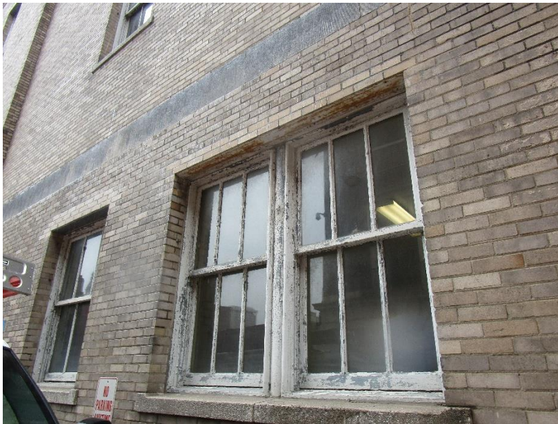
Figure 58. Windows at north elevation of 18 Trinity Street.
