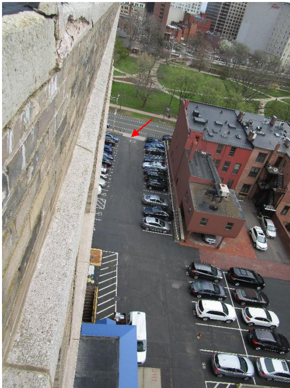
Figure 106. Parking lot. Note storm drain.
