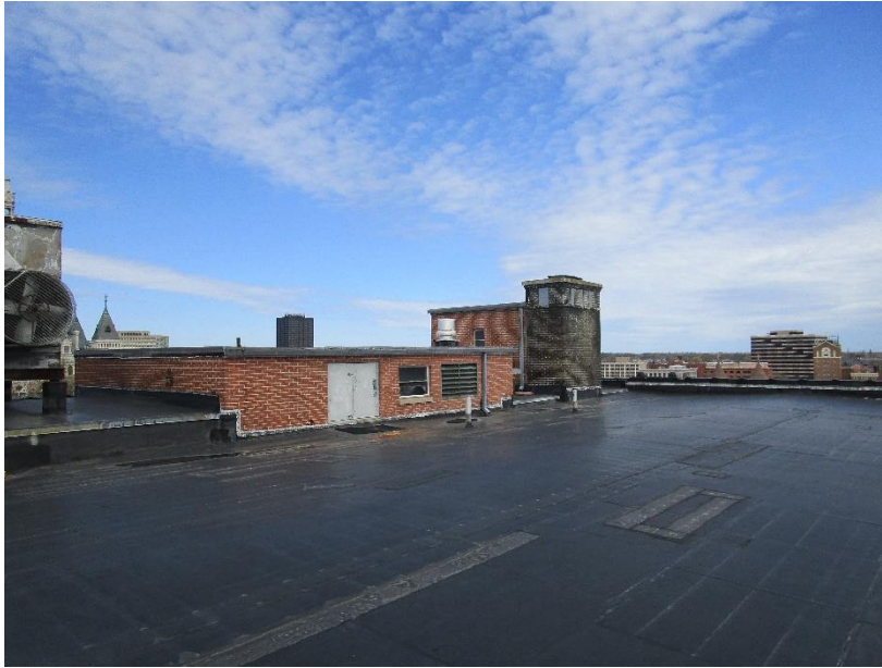
Figure 63. Roof at 18 Trinity Street.
