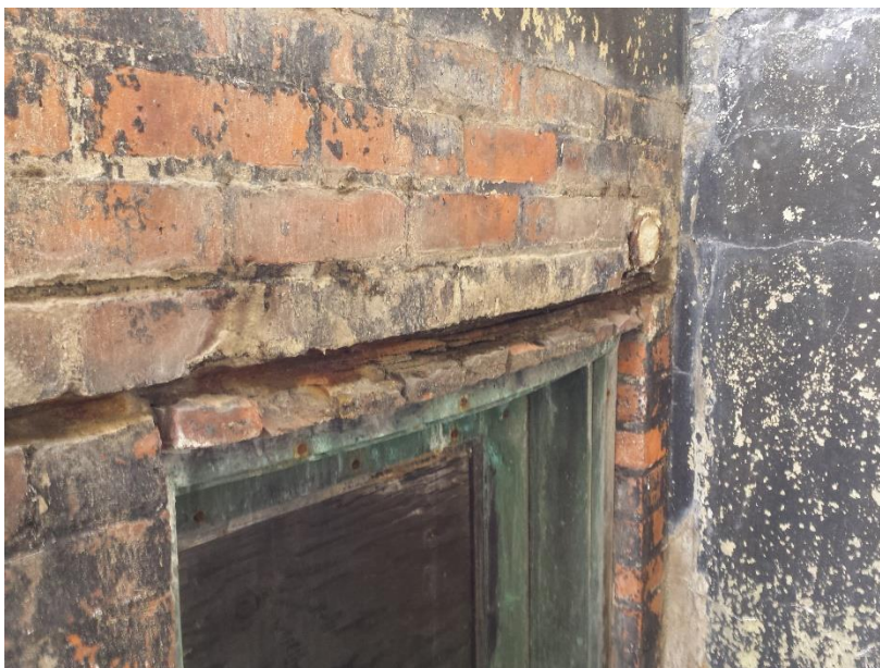
Figure 76. Head at door to vault at 18 Trinity Street.
