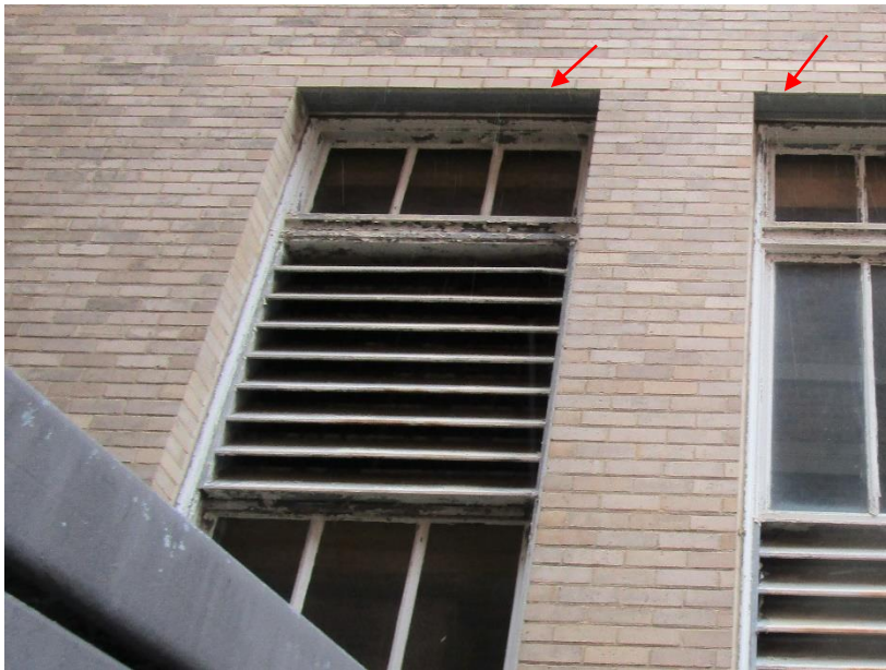
Figure 52. Galvanized steel replacement lintels.
