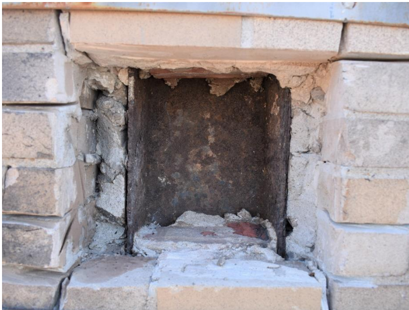
Figure 42. Steel column at the southeast corner of 18 Trinity Street.
