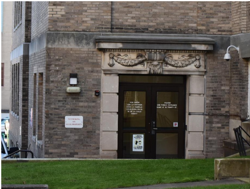
Figure 38. Door and sidelight at northwest entrance to 18 Trinity Street.
