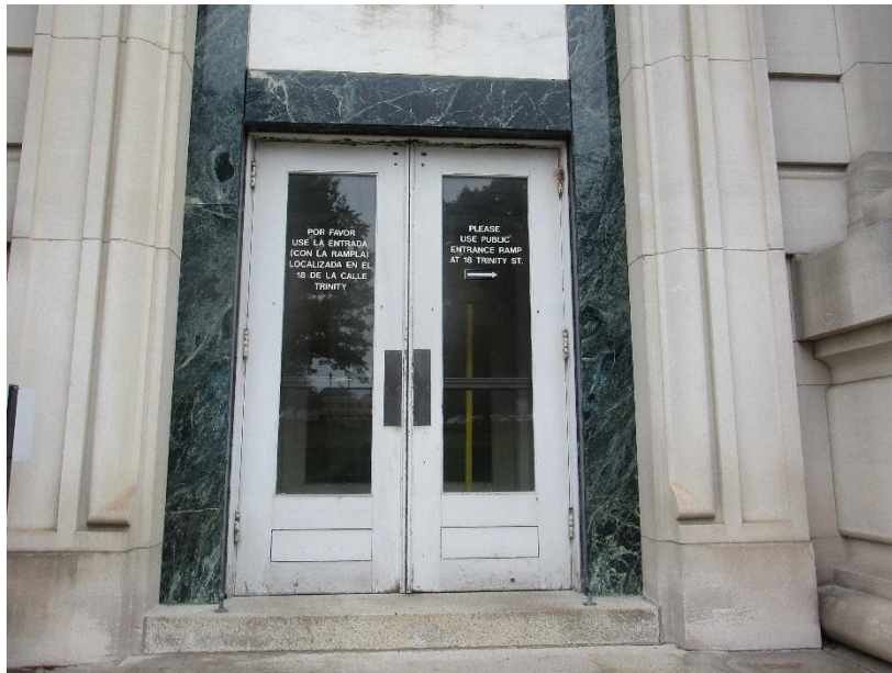
Figure 26. Door at west entrance.
