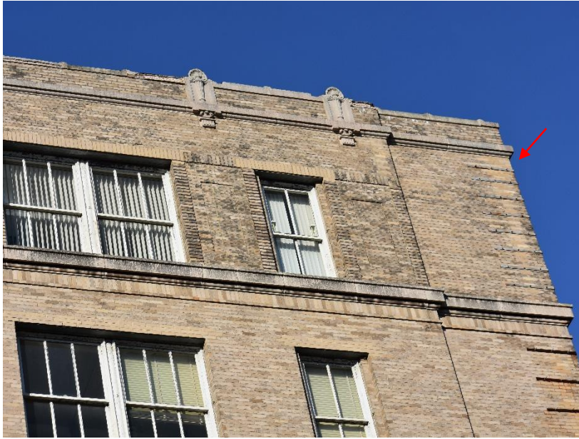
Figure 39. Steel straps at northeast corner of 18 Trinity Street.
