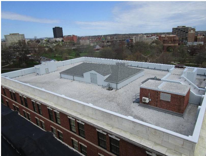
Figure 100. Roof at 30 Trinity Street.
