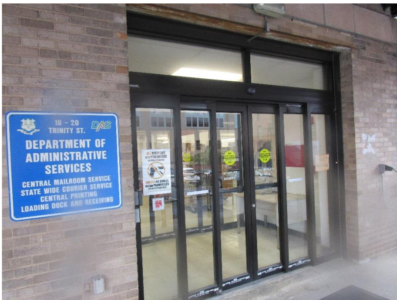
Figure 62. Sliding aluminum/glass doors at loading dock.
