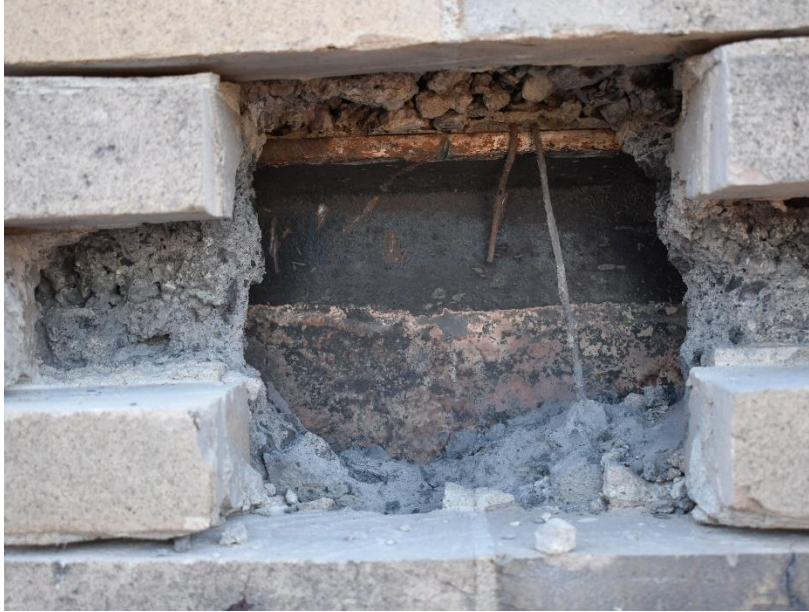
Figure 43. Steel spandrel beam at north elevation.
