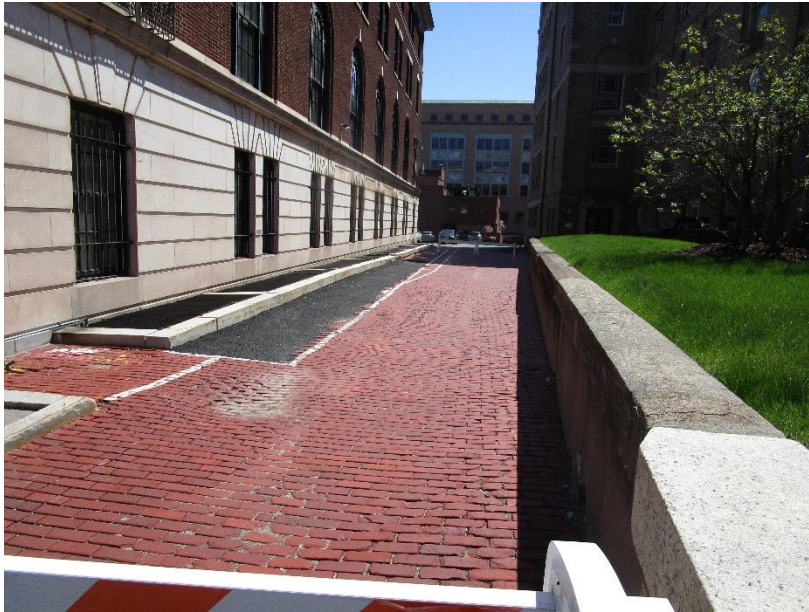
Figure 107. Driveway from Trinity Street to the parking lot.
