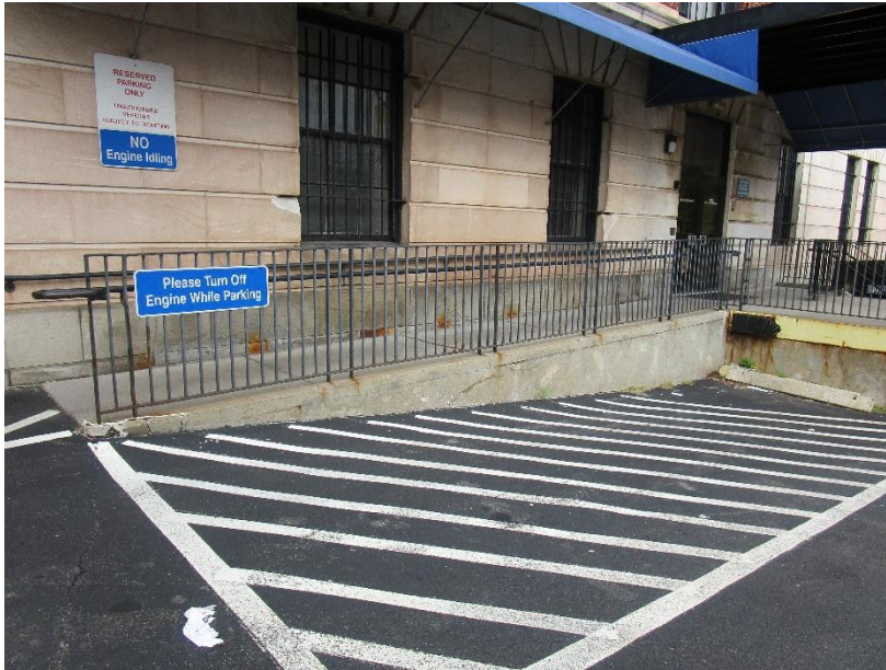
Figure 126. Ramp to east entrance to 30 Trinity Street.
