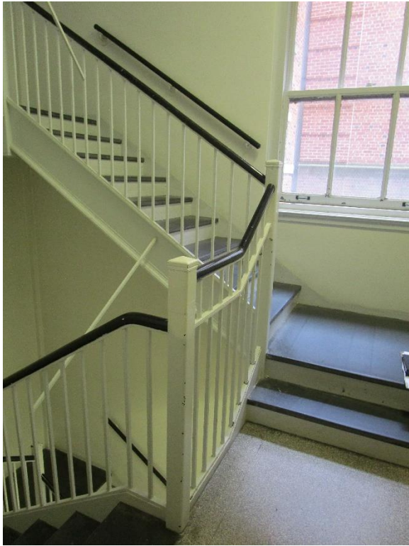
Figure 116. Typical handrails at 18 Trinity Street stairs.
