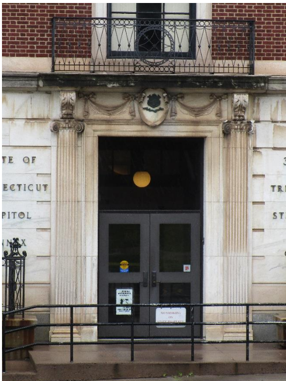
Figure 98. West entrance doors at 30 Trinity Street.
