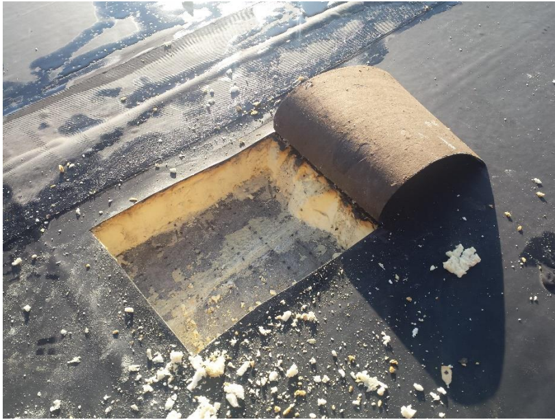
Figure 71. Roof probe at field of roof at 18 Trinity Street.
