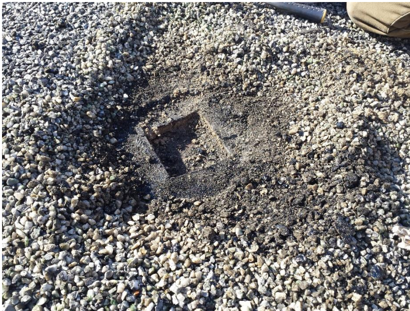
Figure 28. Roof opening at 20 Trinity Street.
