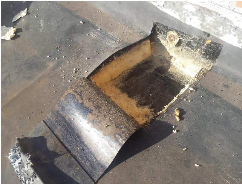
Figure 72. Roof probe at rising wall at 18 Trinity Street.
