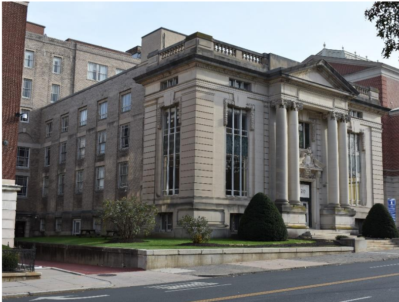
Figure 2. North façade at 20 Trinity Street.
