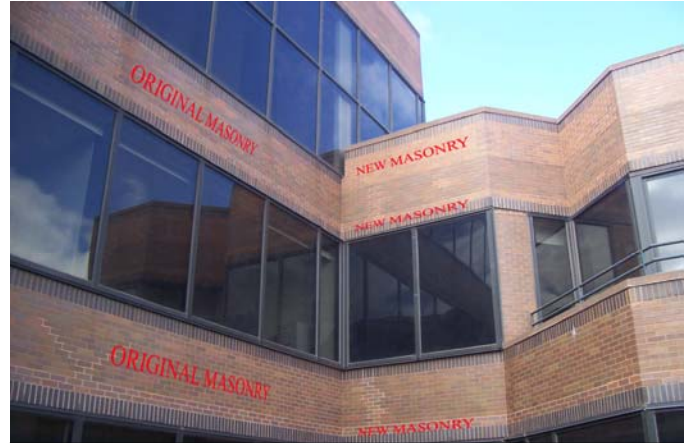
2. Representative Areas of Masonry Repairs Done by Kelly Enterprises (19 th floor)
