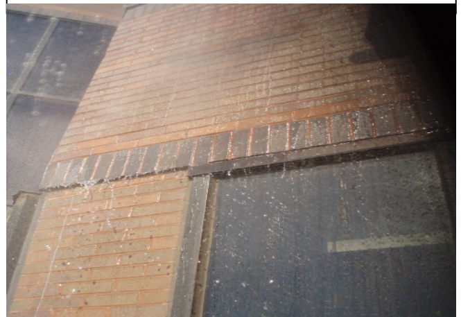
6. Flood Testing (19 th Floor Interior Balcony)
