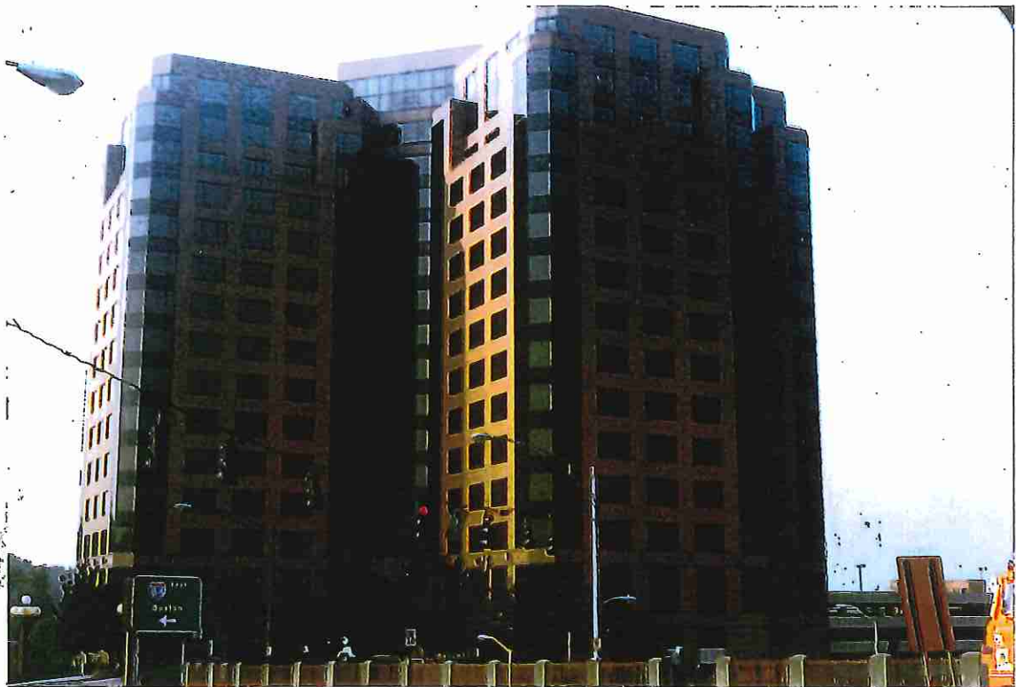
#1 Front view of the building from the northeast, viewed from Sigourney Street ramp to I-84.
