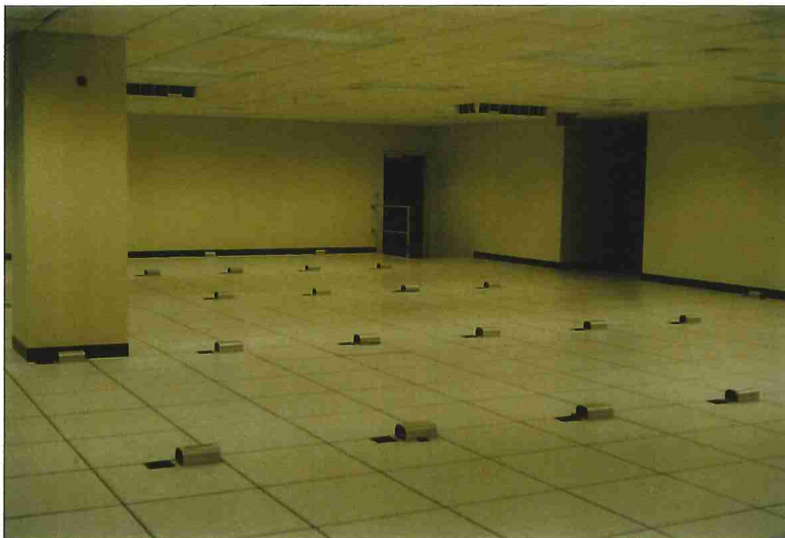
#12 16th floor computer room.
