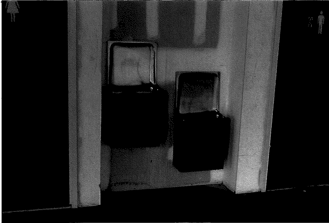
#15 Typical paired drinking fountains. "Accessible" unit is not cantilever design for wheelchair access.
