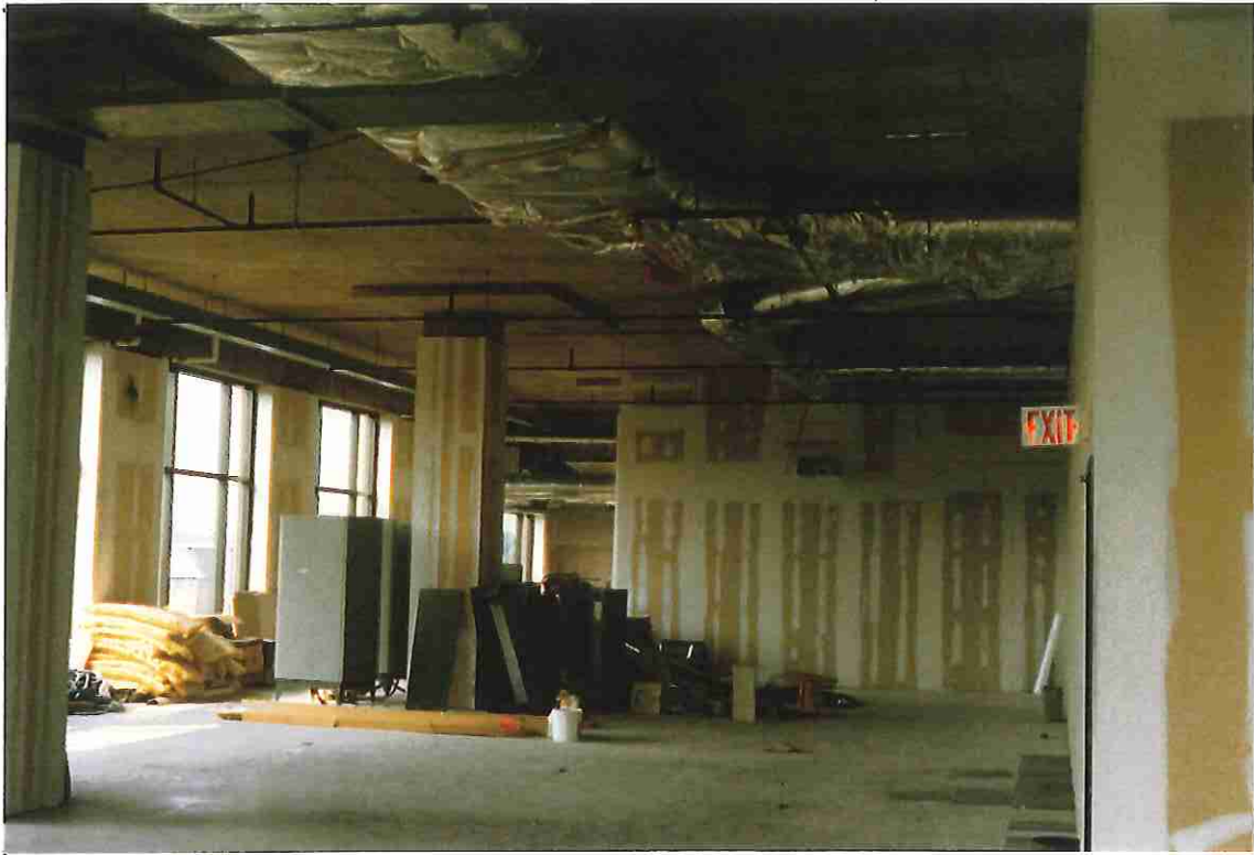
#5 Exposed structural slab in unfinished space on mezzanine level.
