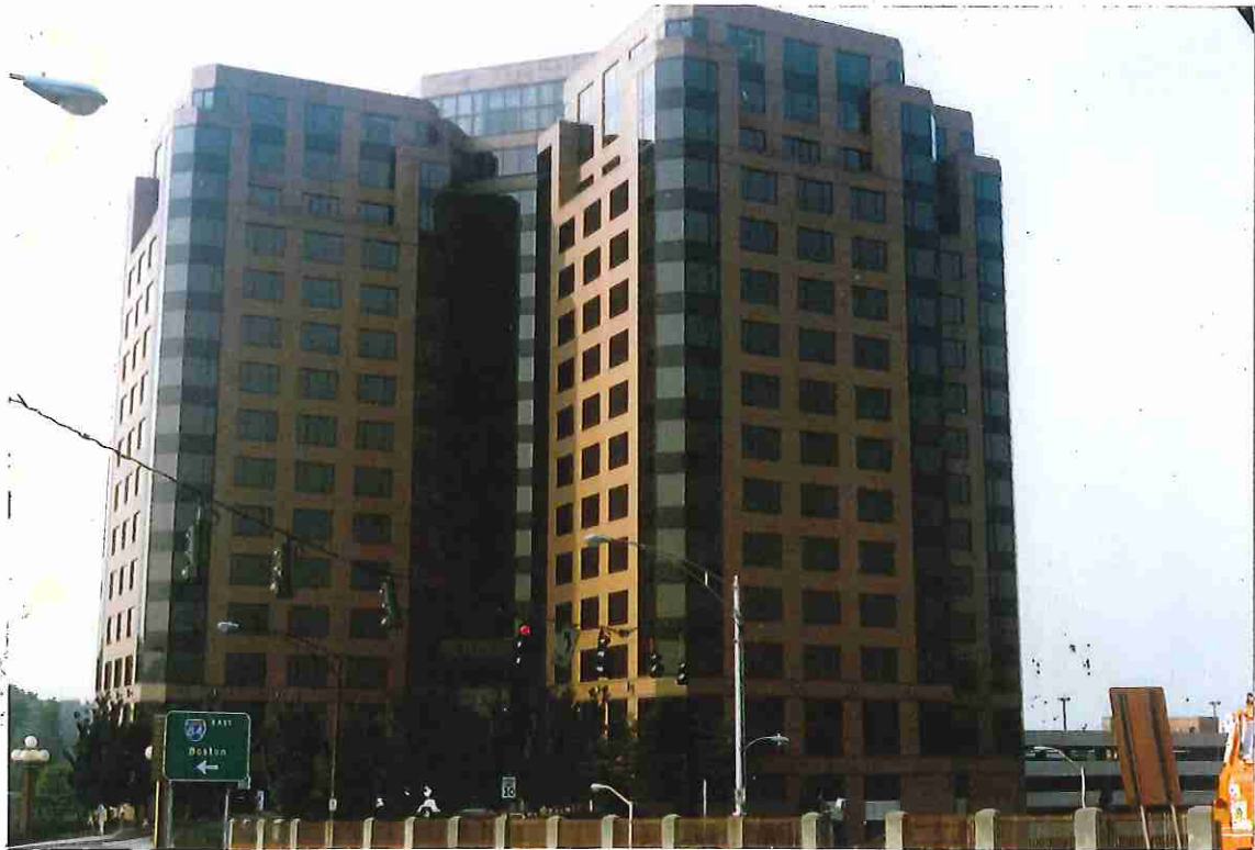
#1 Front view of the building from the northeast, viewed from Sigourney Street ramp to I-84.
