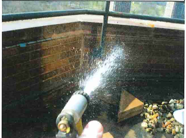
Soaking the Interior Parapet Wall
