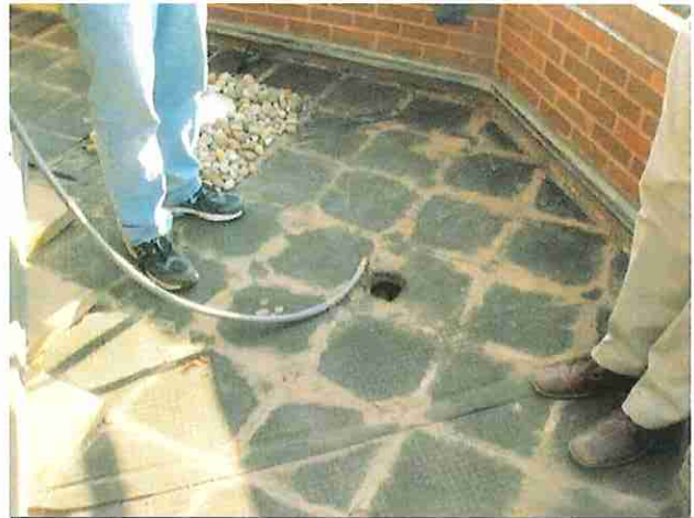
Condition of Roof Membrane
