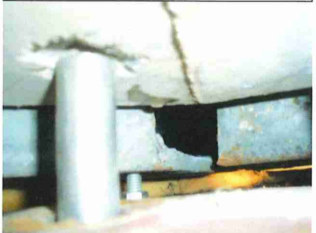
Discontinuous Steel Angle @ Corner (Area where the exterior water infiltrates)
