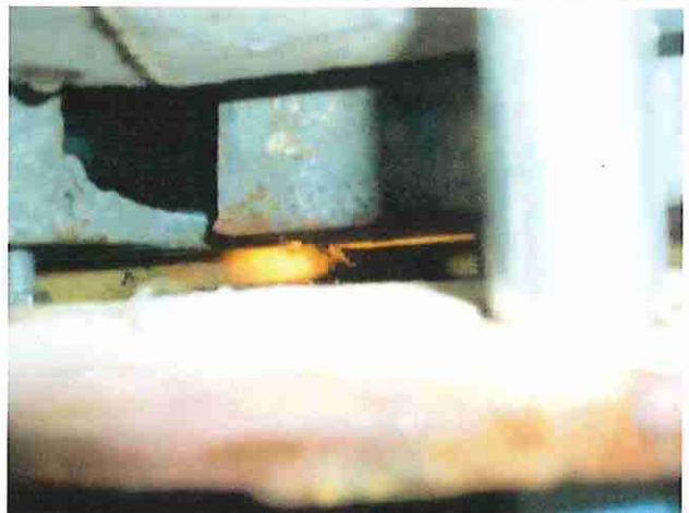
Discontinuous Steel Angle @ Corner (Area where the exterior water infiltrates)
