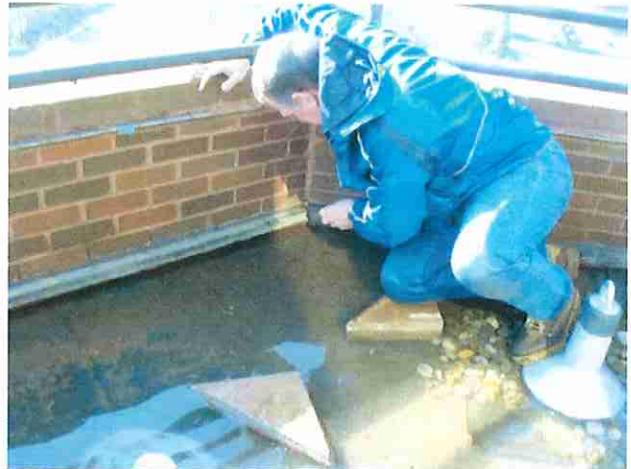
Searching for Leaks above Reglet
