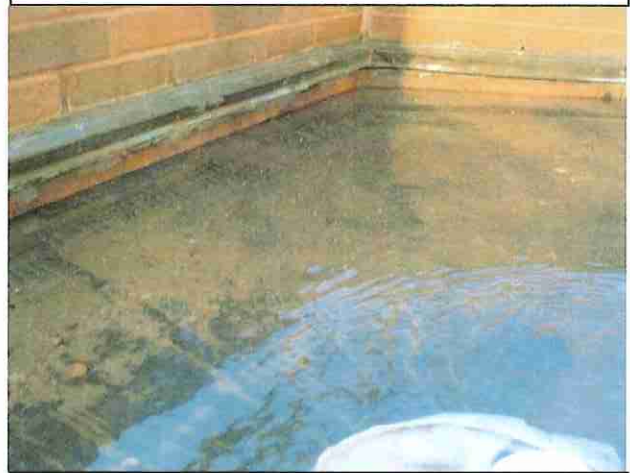
Flooding the Roof Membrane
