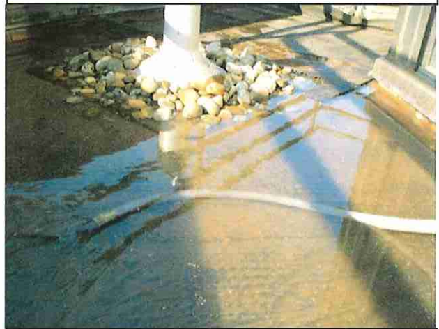
Flooding the Roof Membrane
