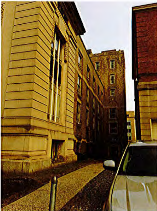
South side 45 windows
