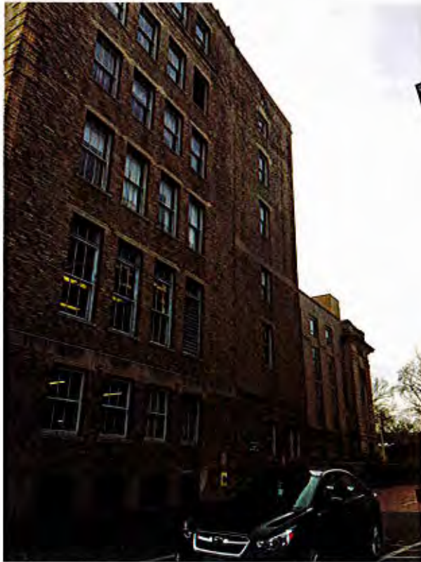
North side 59 windows
