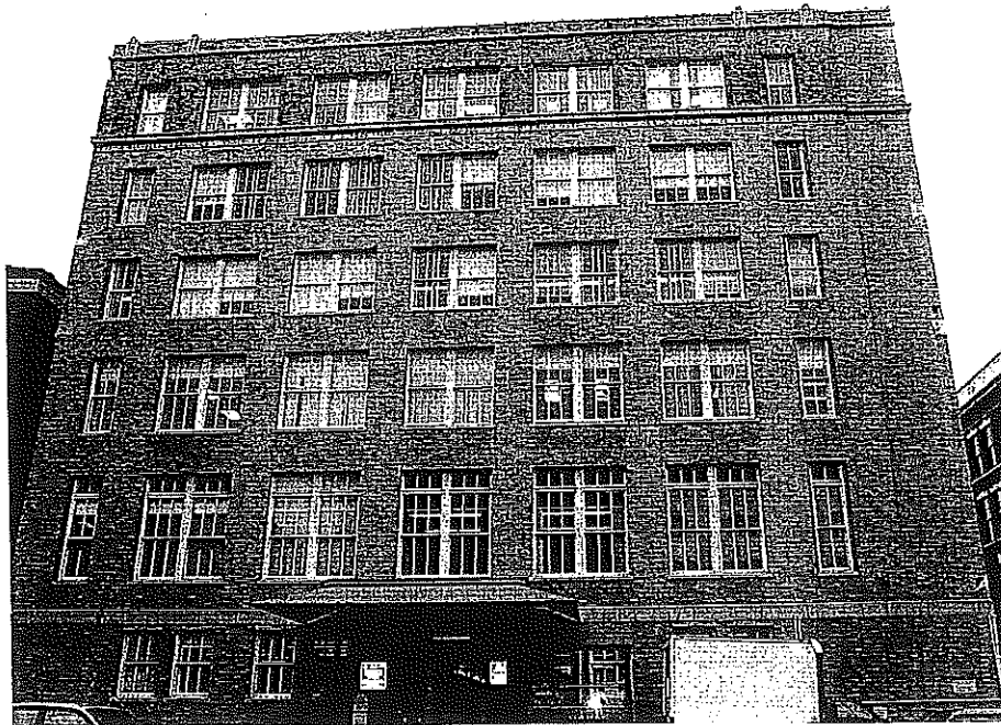
PHOTO# 4 EAST ELEVATION
