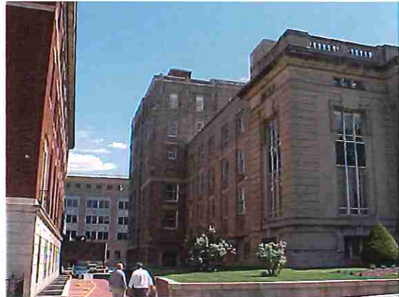
Photo #2: Left side elevation of 3-story portion of building
