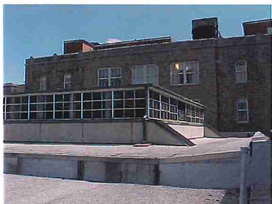
Photo #6: Front elevation of 6-story portion of building
