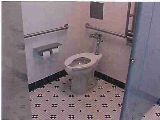
Photo #39: ADA accessible bathroom
