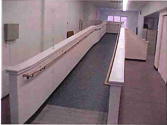
Photo #43: New ADA accessible ramp
