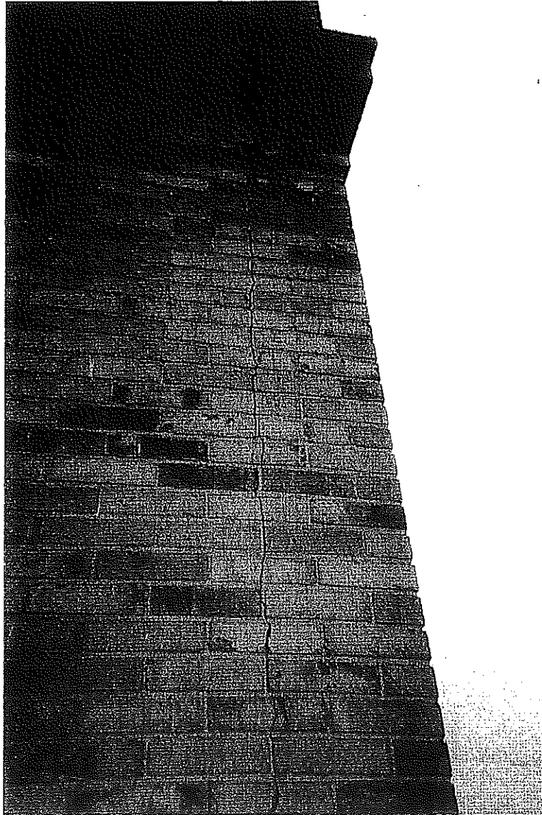
PHOTO #24 CONTINUOUS VERTICAL CRACK FROM THE TOP OF THE PARAPET DOWN TO THE FOURHT FLOOR OF SOUTHEAST CORNER. NOTE, BOTTOM SECTION OF THE PRECAST CONCRETE CORNICE FELL OFF.
