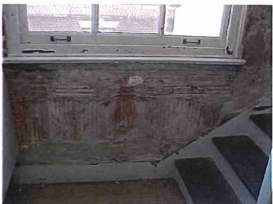
Photo #30: Removed plaster wall finish for north stairwell
