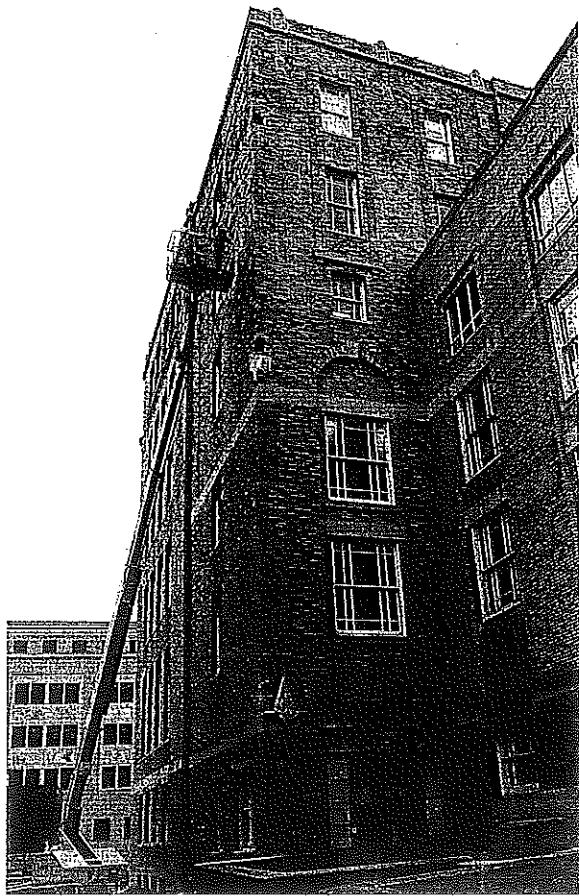
PHOTO# 1 NORTHWEST CORNER
