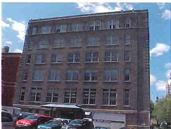
Photo #5: Rear elevation of building
