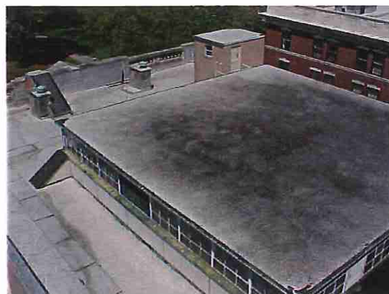
Photo #17: Roof overview at 3-story portion of building
