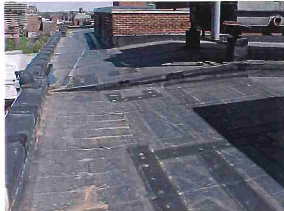
Photo #16: Rubber membrane roof overview at 6-story portion of building
