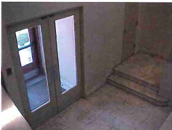
Photo #35: Original main lobby overview
