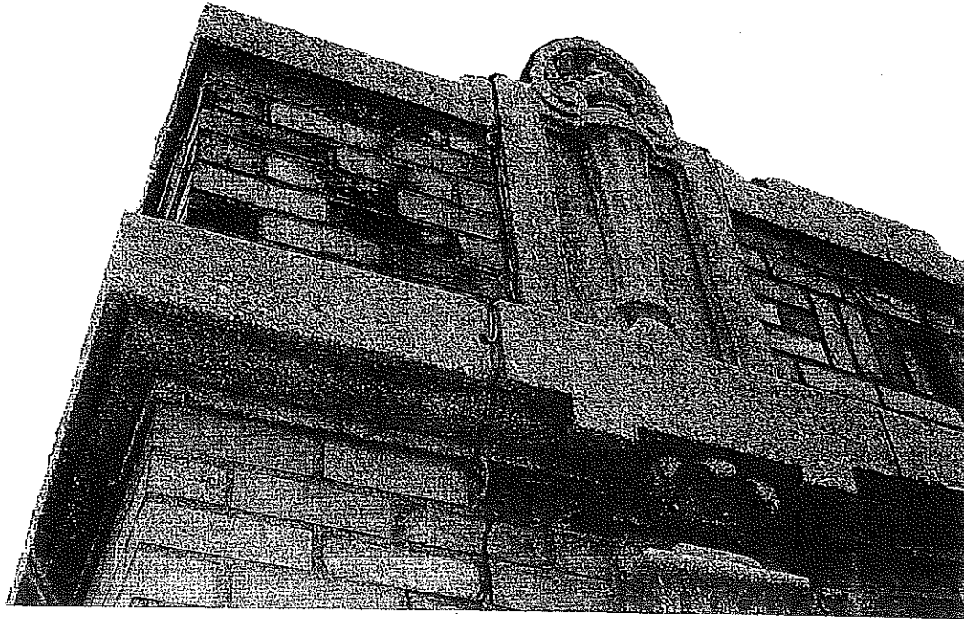
PHOTO #26 PRECAST CONCRETE COPING, DECORATIVE ORNAMENTS AND CORNICES. CAULKING IS MISSING. NOTE VERTICAL CRACK FROM PARAPET AT NORTHEAST CORNER.
