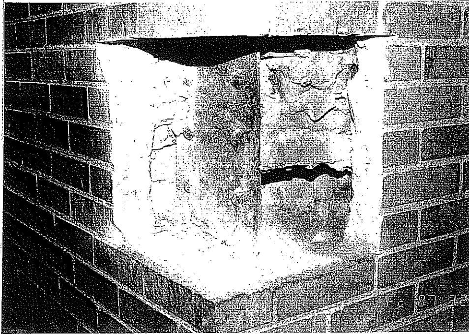
PHOTO# 16 SOUTHEAST CORNER – EXPOSED COLUMN.
