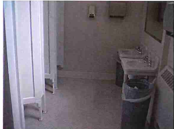
Photo #38: Typical restroom interior
