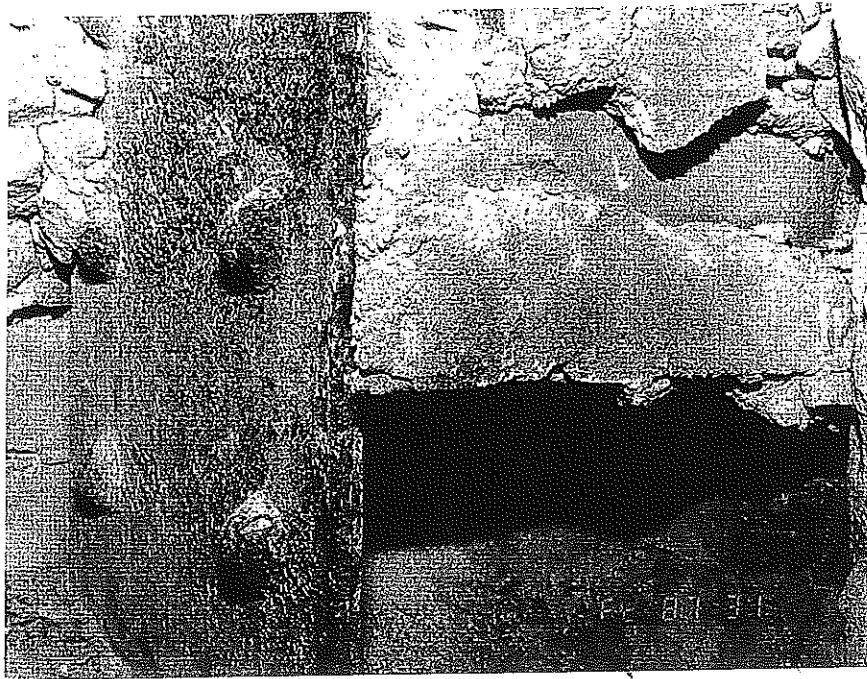
PHOTO# 17 SOUTHEAST CORNER – PHOTO# 16 CLOSE UP.
