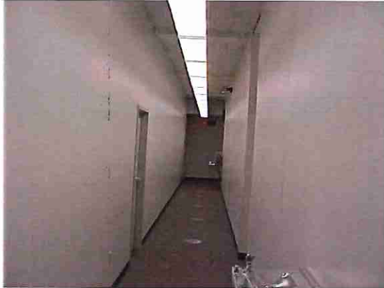
Photo #37: Typical common corridor interior
