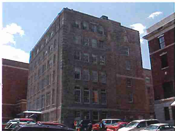
Photo #4: Left side elevation of 6-story portion of building
