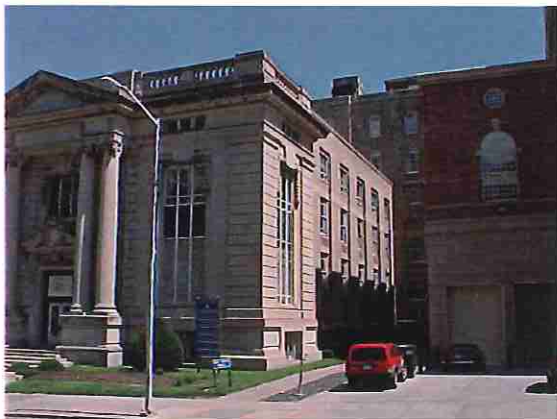
Photo #3: Right side elevation at 3-story portion of building
