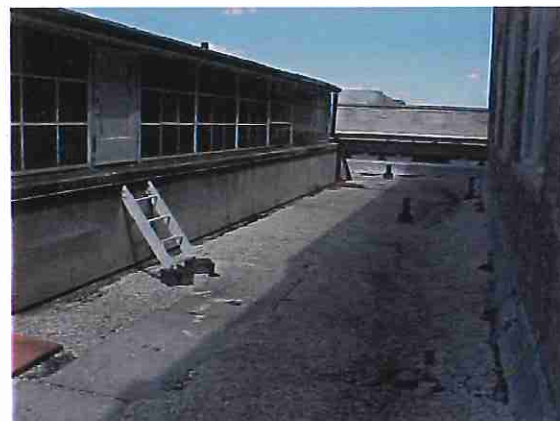
Photo #18: Built-up roof overview at 3-story portion of building
