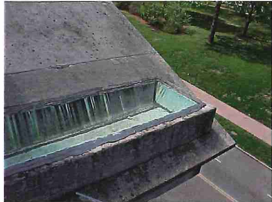
Photo #20: Stone roof slab with built-in gutter at front entry porch
