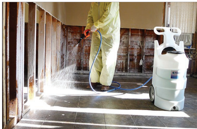
Figure 2. Pump-up or motorized foam generators can apply a wide range of cleaning chemicals
