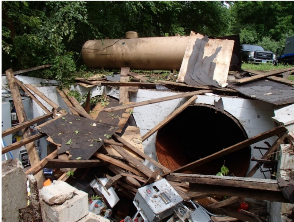
Fig. 1 Catastrophic hydropneumatic tank explosion in June 2015 that left 3,000 CWS customers without water and precipitated the passage of the new asset and fiscal plan with prioritized hydropneumatic tank assessment requirement for small CWS.
