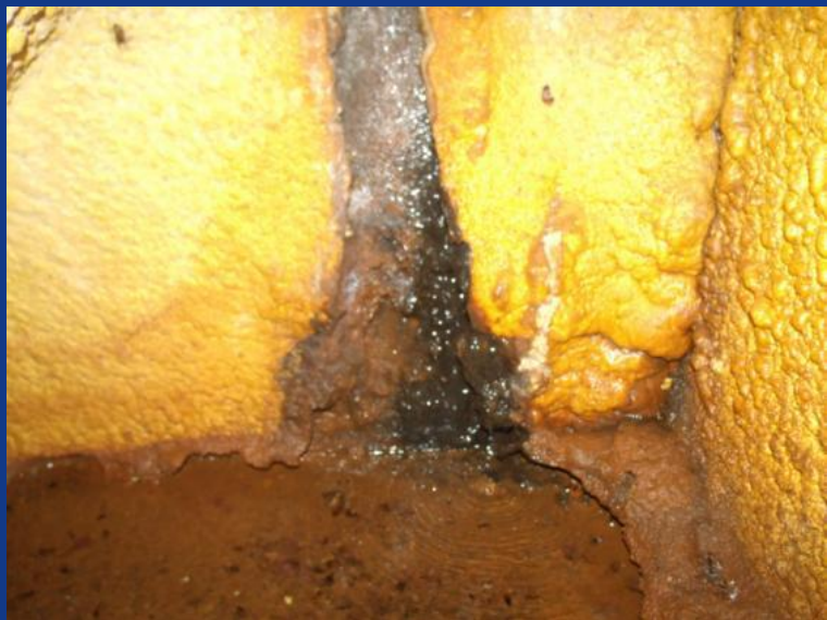
Foundation wall leaking water
