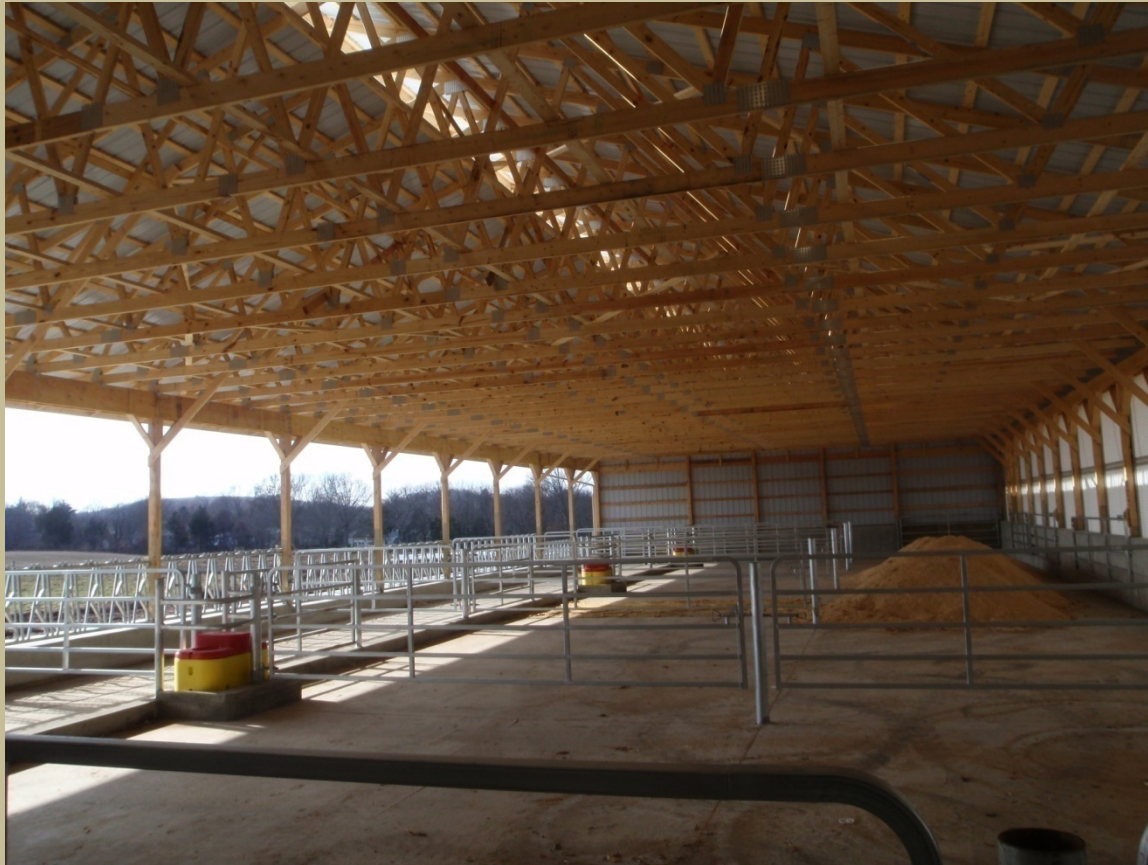
Covered Manure Storage
