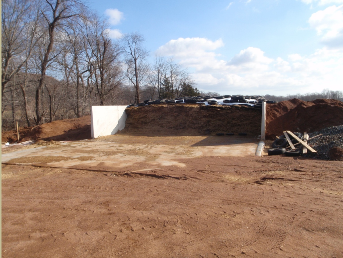
COVERED BUNKER SILO
