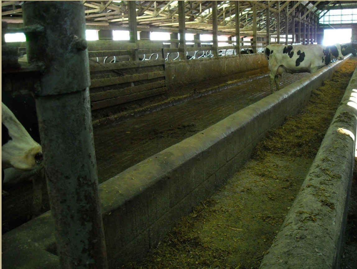
Roofed Heavy Area
