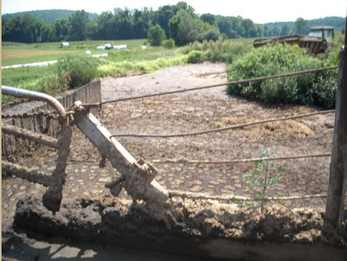
OVERFLOWING WASTE STORAGE
