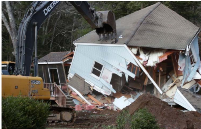
Demolition of a flooded house on River Trail Road, Southbury CT.
