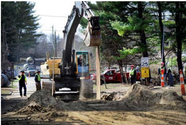
Photo from The News-Times of the drainage project construction
