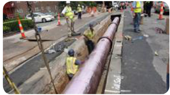
Water Main Installation Photo by DPH.
