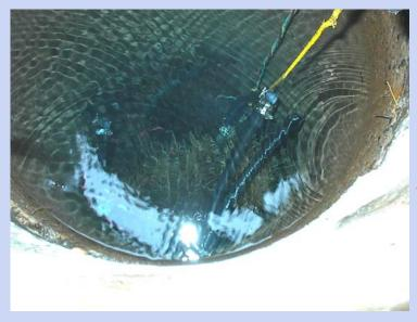
Additional photographs of this dug well also indicate that the side walls are not four inches thick. Dug wells rarely meet the criteria specified in RCSA Section 19-13-BSIf (b).
