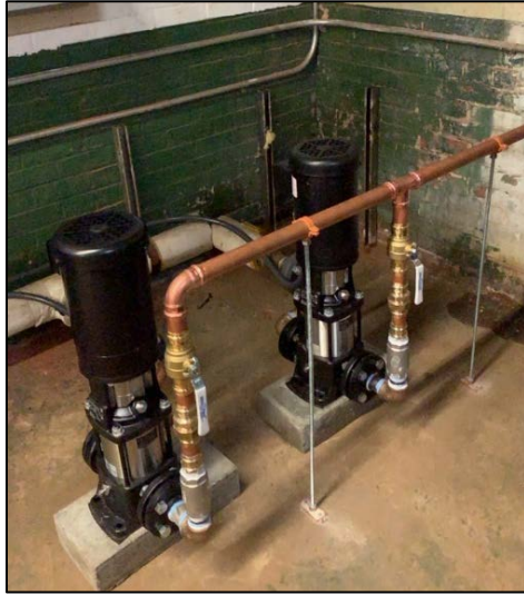
Fig. 5 New booster pumps and tank which were installed at the Housatonic Regional School District No. 1 small public water system to replace aging infrastructure. The project was funded by the DWSRF.
