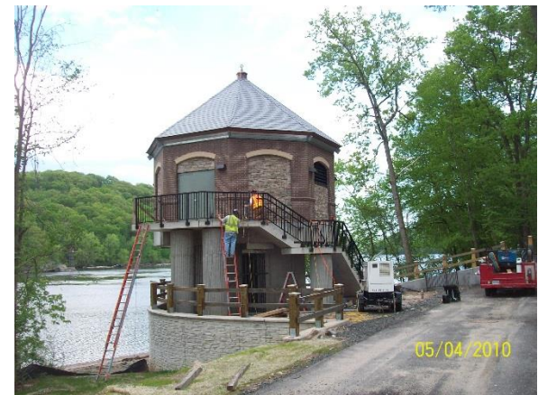
Photo of Collector Well by MMI
