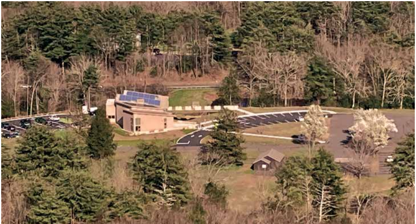
A view from above of the new Western District Headquarters building at Black Rock State Park in Watertown. The roof features solar panels to help reduce energy use.
