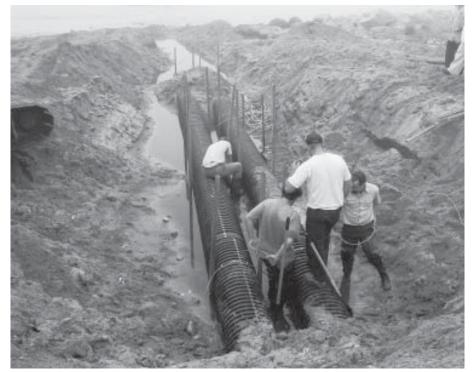
Workers install two culverts in East Lyme to restore a tidal pond that had previously converted to a freshwater pond.
