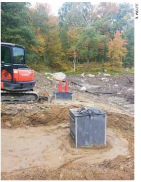
Compaction has been completed on two inline water control structures.
