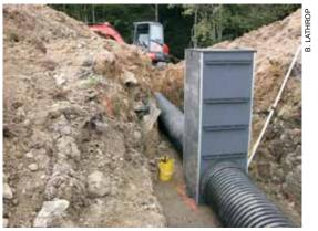
View of a 24-inch diameter ADS N-12 pipe attached to an eight-foot Agri-Drain inline water control structure.
