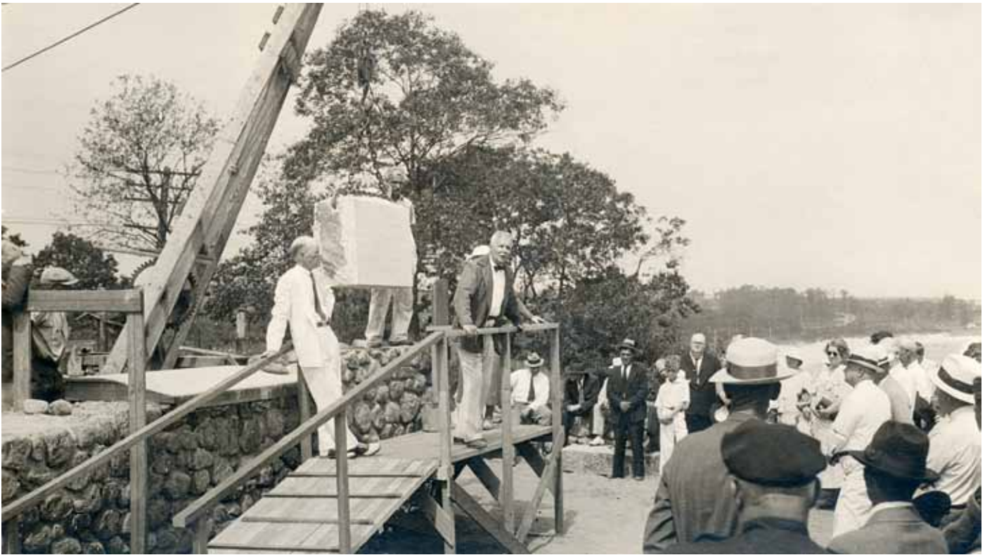
With the stone foundation of Rocky Neck State Park's 330-foot long pavilion near completion, speeches accompanied the June 1935 laying of the ceremonial cornerstone. The park's half-mile long beach and 250 adjoining acres provided the public with a generous shoreline park on Connecticut's southeastern coast.
