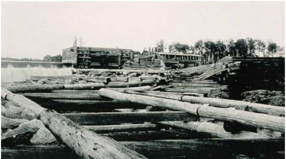
**Early fishways on the river, like this one near Turners Falls, Massachusetts, were constructed from logs but located in a way that made it difficult for fish to find and use.**
