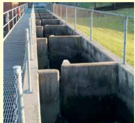
The Rainbow Fishway on the Farmington River is the only vertical slot fishway in the state.
