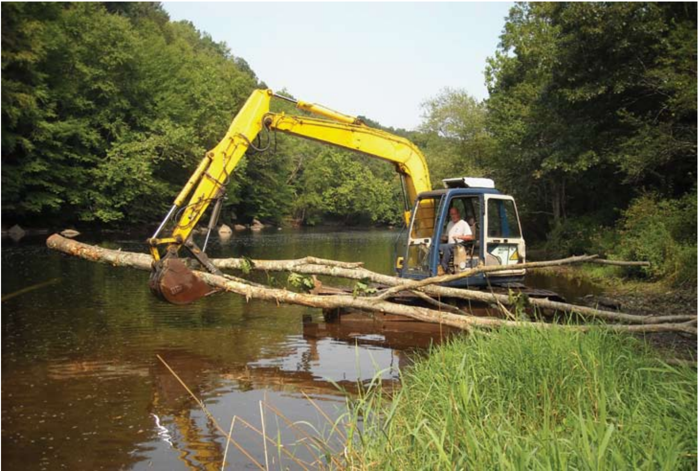
Donnie Hargreaves of the DEP's Wetlands Habitat and Mosquito Management Program constructs a log jam in the Shetucket River to create "Large Woody Habitat."
