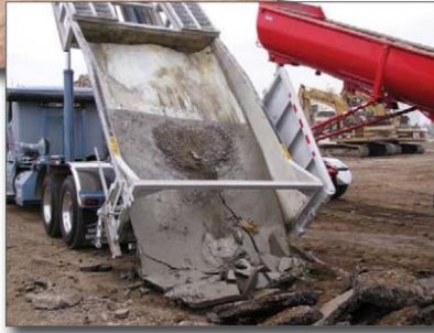
Figure 15. Delivering hardened Concrete to a recycler
