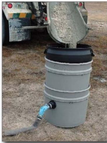
Figure 3. Concrete washout filter
