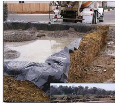
Figure 9. Hay bale and plastic washout pit
