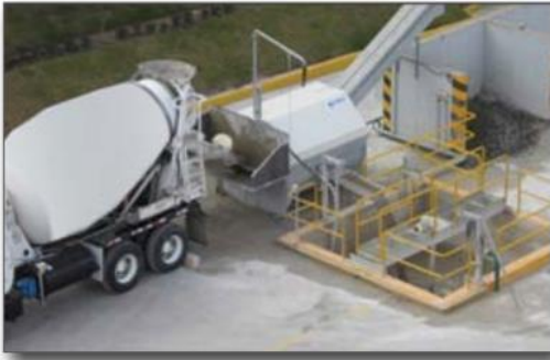
Figure 5. Ready mixed truck washing out into a reclaimer
