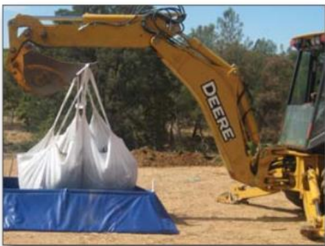
Figure 12. Extracting the concrete solids or gelled washwater
