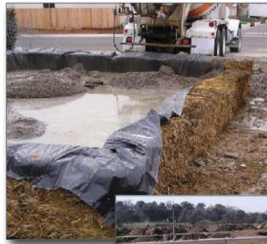
Figure 9. Hay bale and plastic washout pit
