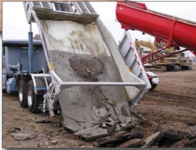
Figure 15. Delivering hardened concrete to a recycler
