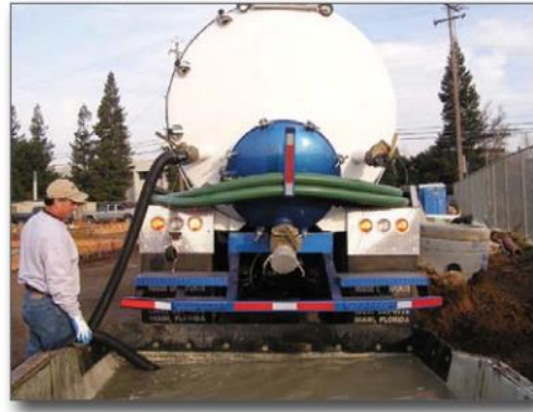
Figure 4. Vacuuming washwater out of a washout container for treatment and reuse
