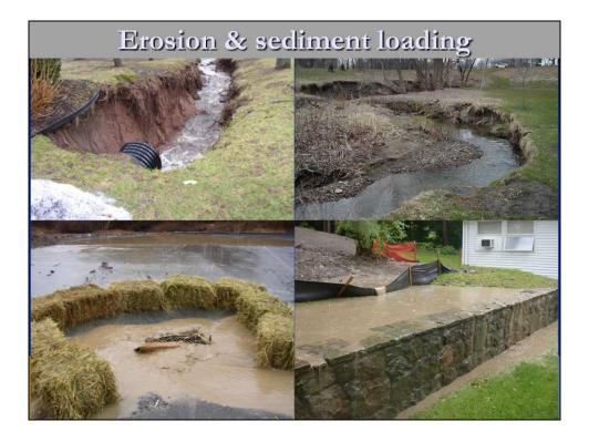
The first two pictures demonstrate the potential for stream bank erosion due to high flow. In the left side, you can see the pipe depositing water into the stream channel. The bottom two show how solids can run off from barren sites, particularly construction sites, and into water bodies. Note that in the lower left picture barrier of hay bales has been placed to filter sediment. However, the system is obviously failing.
